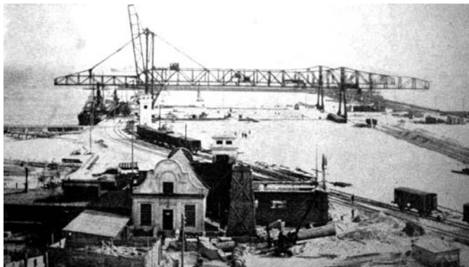
The works of the building, of simple and cheap construction, called "Provisional Naval and Fishing Harbours" started at the end of 1920.
