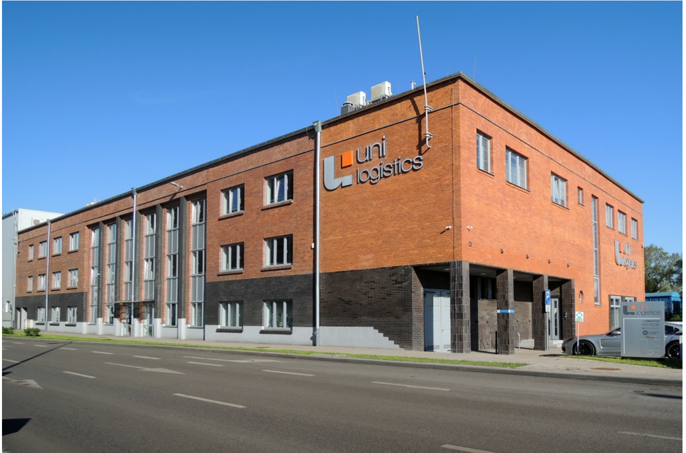
Former “Bananas” Ripening Room, Warehouse and Cold store in the port of Gdynia, after rebuild and expansion of its original structure, view from Polska street. (© Anna Orchowska-Smolinska, 2018)
