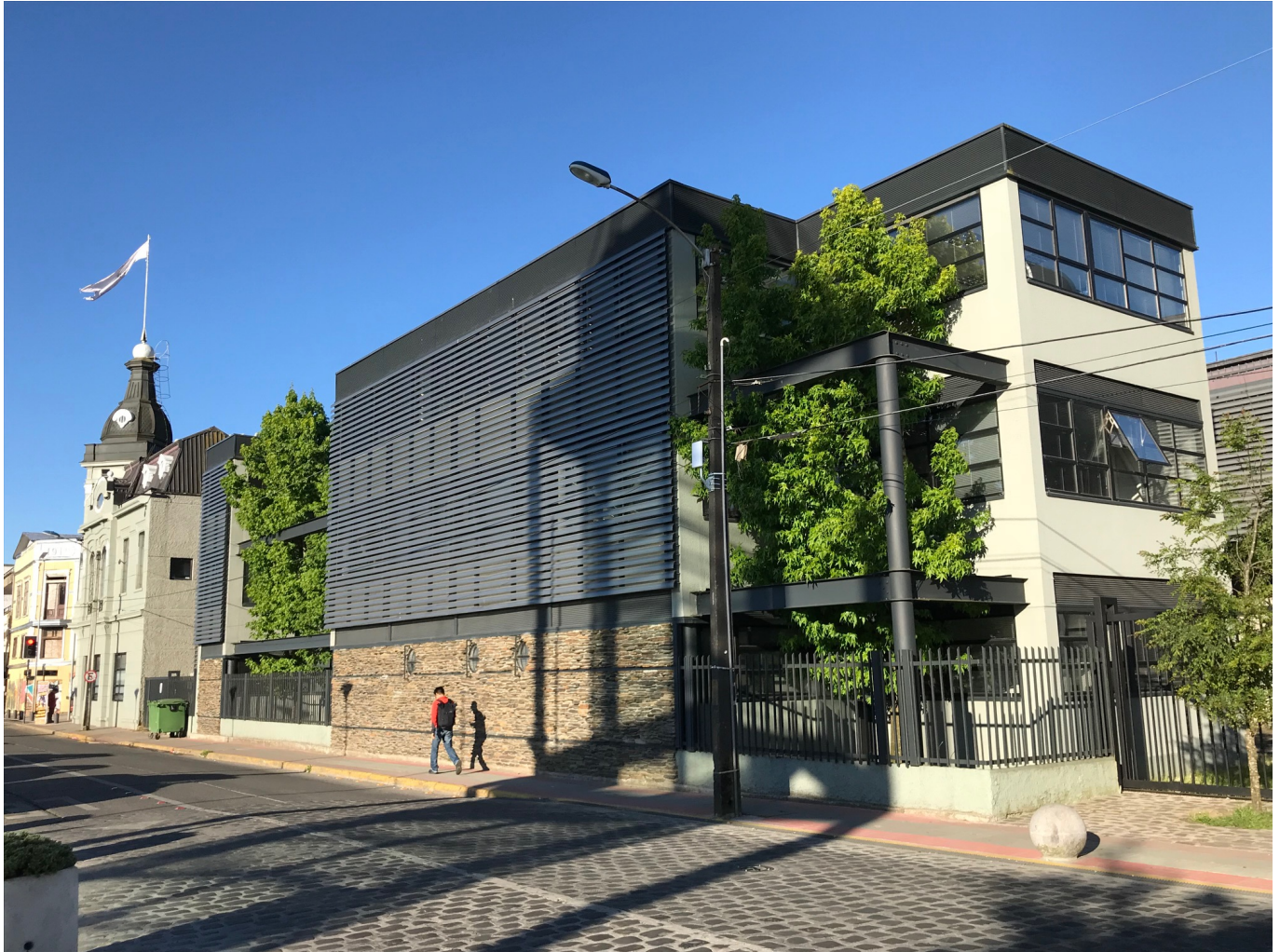
The Glaciology Building facing the river next to the Schuler House. (© F. Basilio, 2017).
