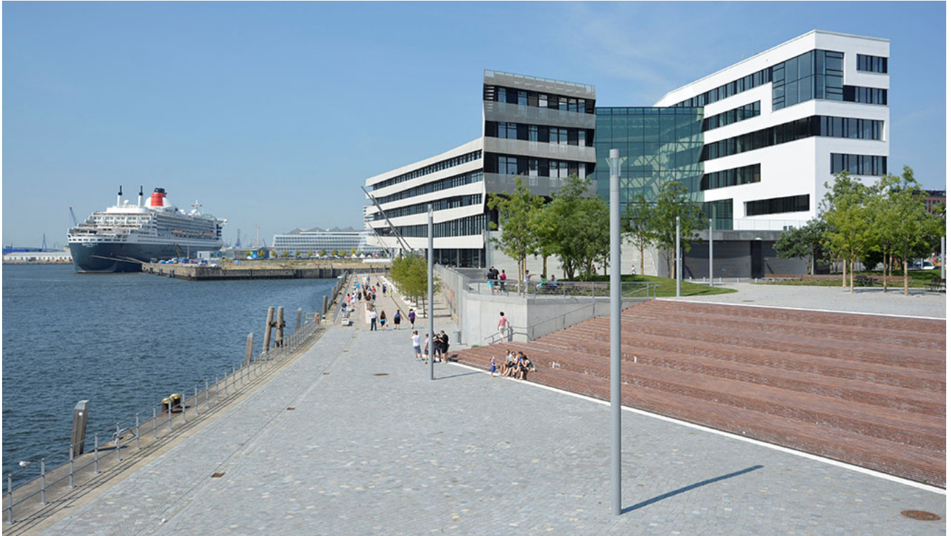
The new building of the Hafencity University on the waterfront in Hamburg. (Source: ELBE&FLUT; Hafencity Hamburg GmbH)
