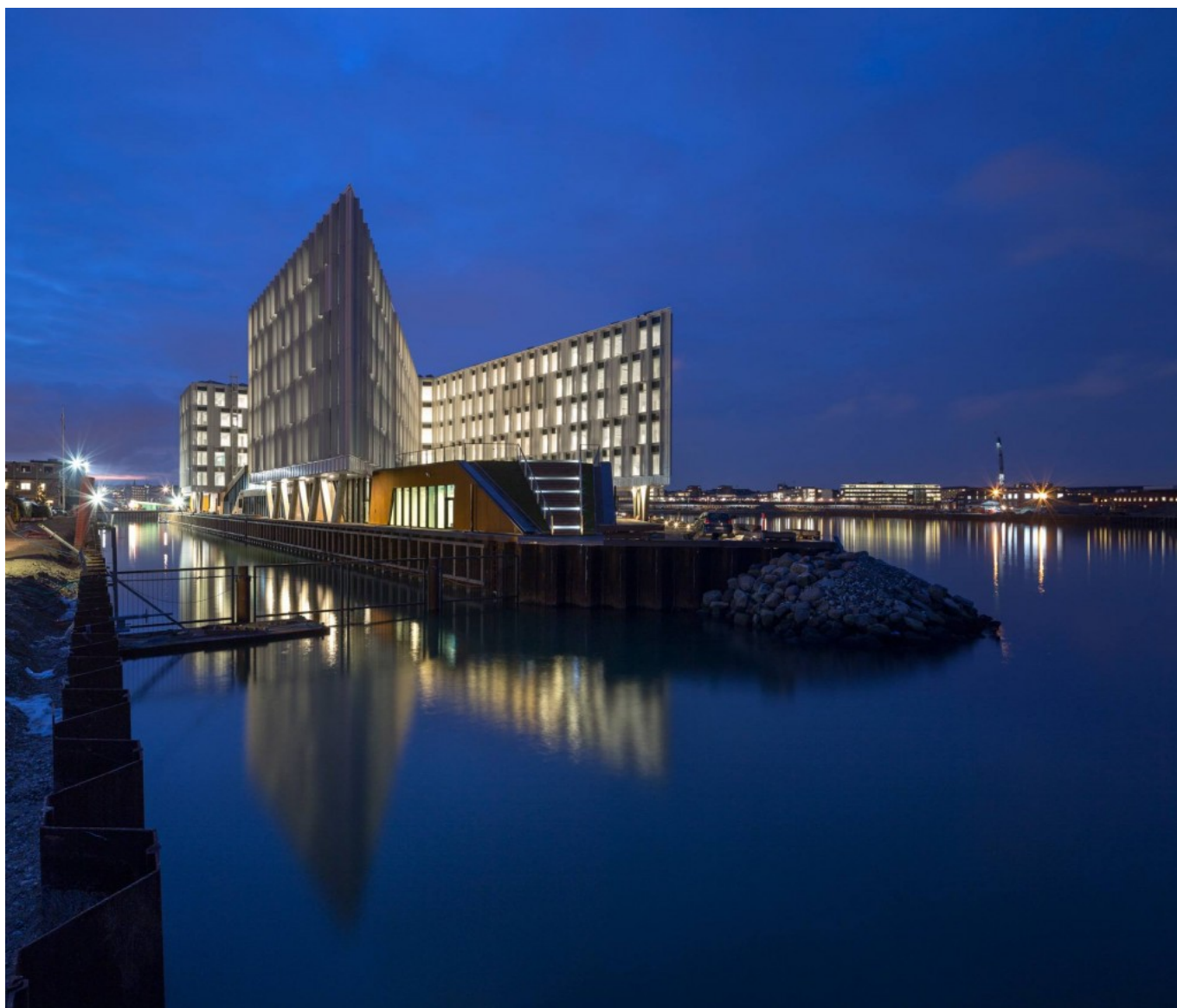
UN City, Copenhagen, Denmark
