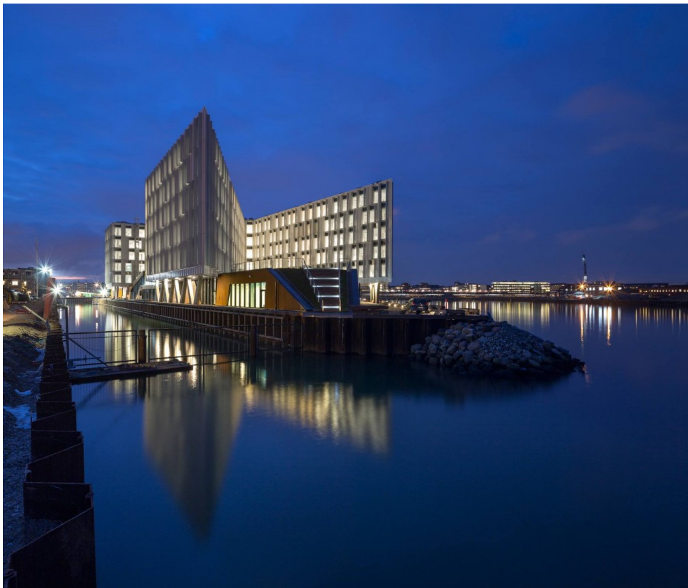
UN City, Copenhagen, Denmark
