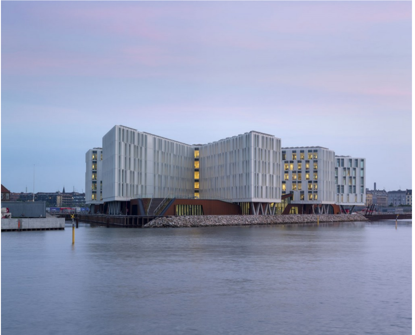
UN City, Copenhagen, Denmark
