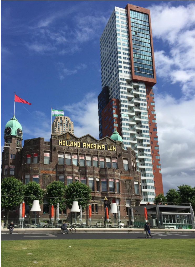
Hotel New York, renovation of the nineteenth century building Holland-Amerika lijn, Rotterdam, Wilhelminapier.
