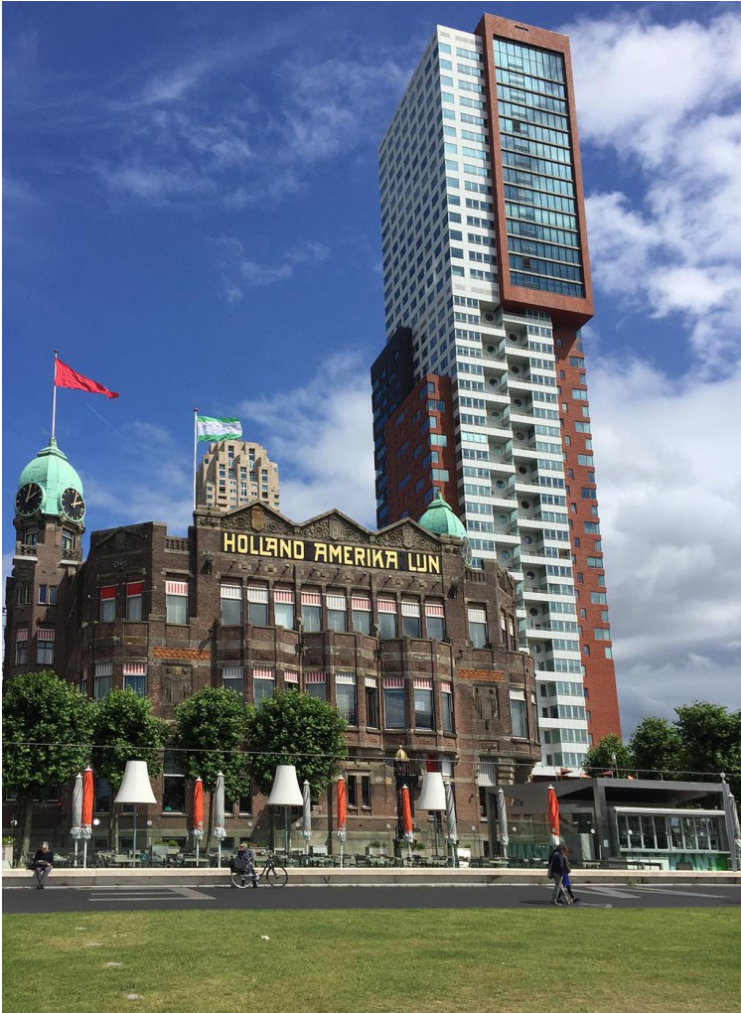
Hotel New York, renovation of the nineteenth century building Holland-Amerika lijn, Rotterdam, Wilhelminapier.
