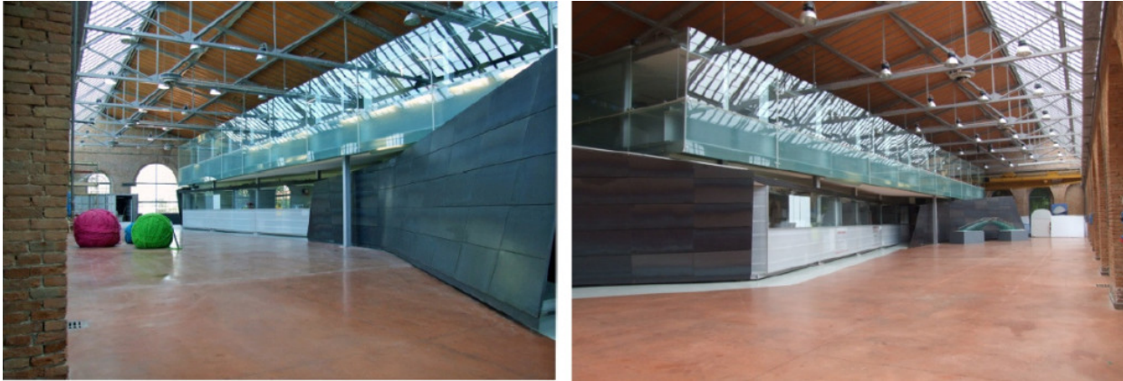
Thetis s.p.a. headquarter (Lamierini building), project: Iginio Cappai and Pietro Mainardi architects (1° fase, 1989/1997), Thetis s.p.a. and Arch. Alberto Cecchetto (2° fase, 2001/2002). Copyright: Arch. Claudio Menichelli.
