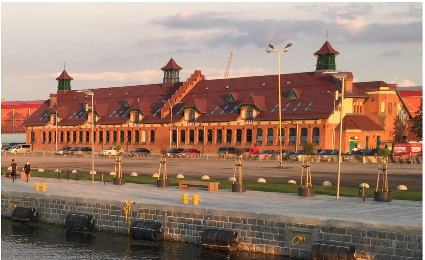
View of Euroregion Cultural Center after adaptation. (Source: photo by Z. Paszkowski)
