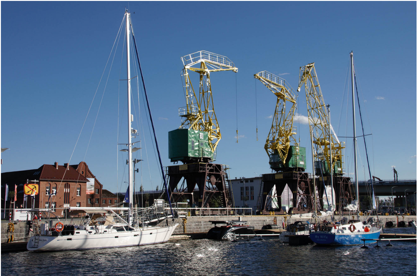
Renovated original cranes called “cranesaurus” in Łasztownia in Szczecin. (Source: photo by Z. Paszkowski)
