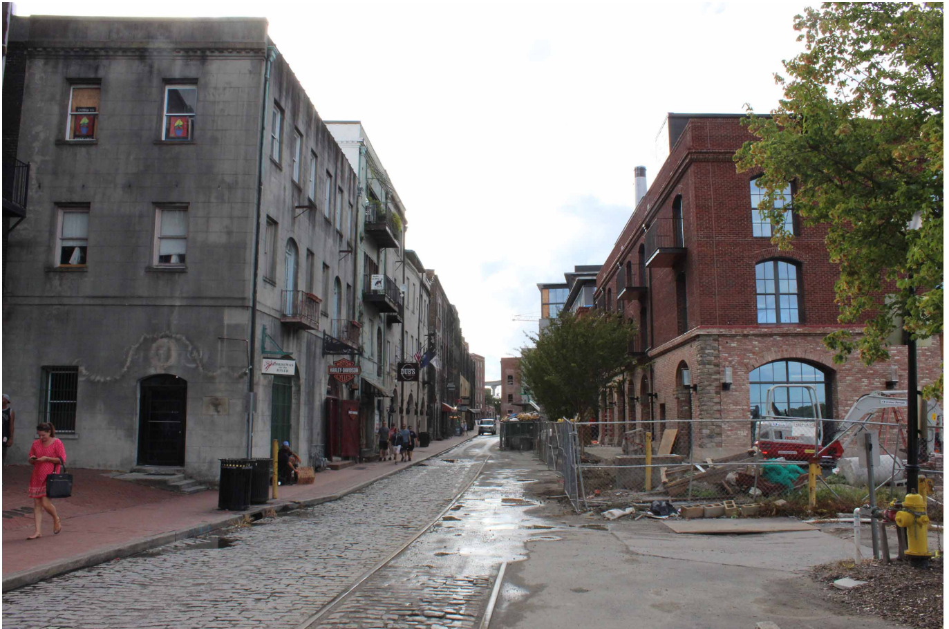
View of the new Power plant Hotel under Construction on River Street East. (Photo by Author)
