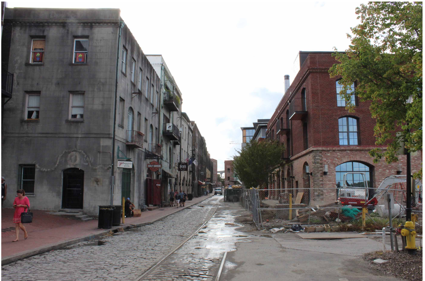
View of the new Power plant Hotel under Construction on River Street East. (Photo by Author)
