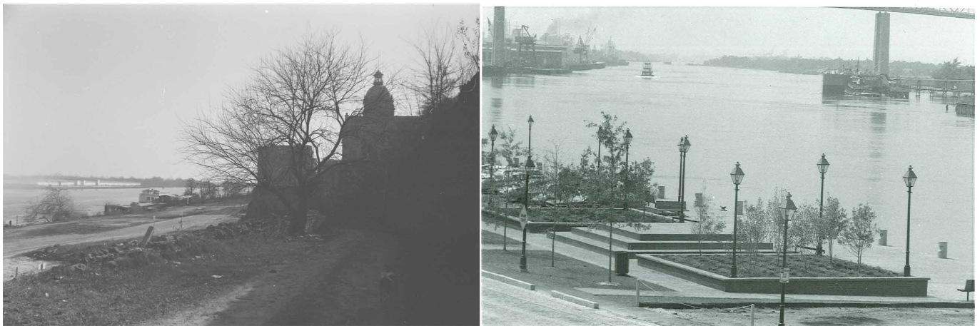
1973. Left: View of the demolition below City Hall; Right: View of the finished Rousakis looking up river. (Record Series 1121-056, Riverfront Urban Renewal Project designed by Gunn & Meyerhoff A.I.A., Architects Courtesy of the Municipal Archives).
