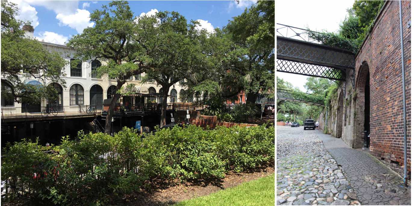
Left: View of Stoddards Range from Bay Street, Right: Cluskey Vaults facing east. (Photos by Author)
