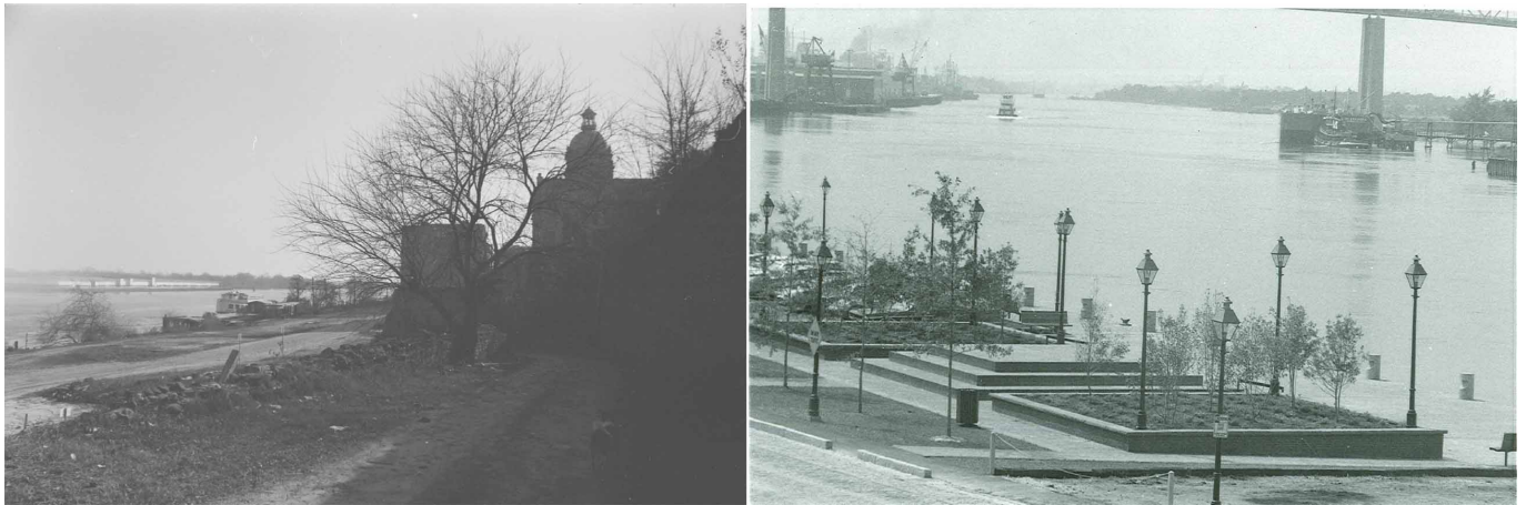
1973. Left: View of the demolition below City Hall; Right: View of the finished Rousakis looking up river. (Record Series 1121-056, Riverfront Urban Renewal Project designed by Gunn & Meyerhoff A.I.A., Architects Courtesy of the Municipal Archives).
