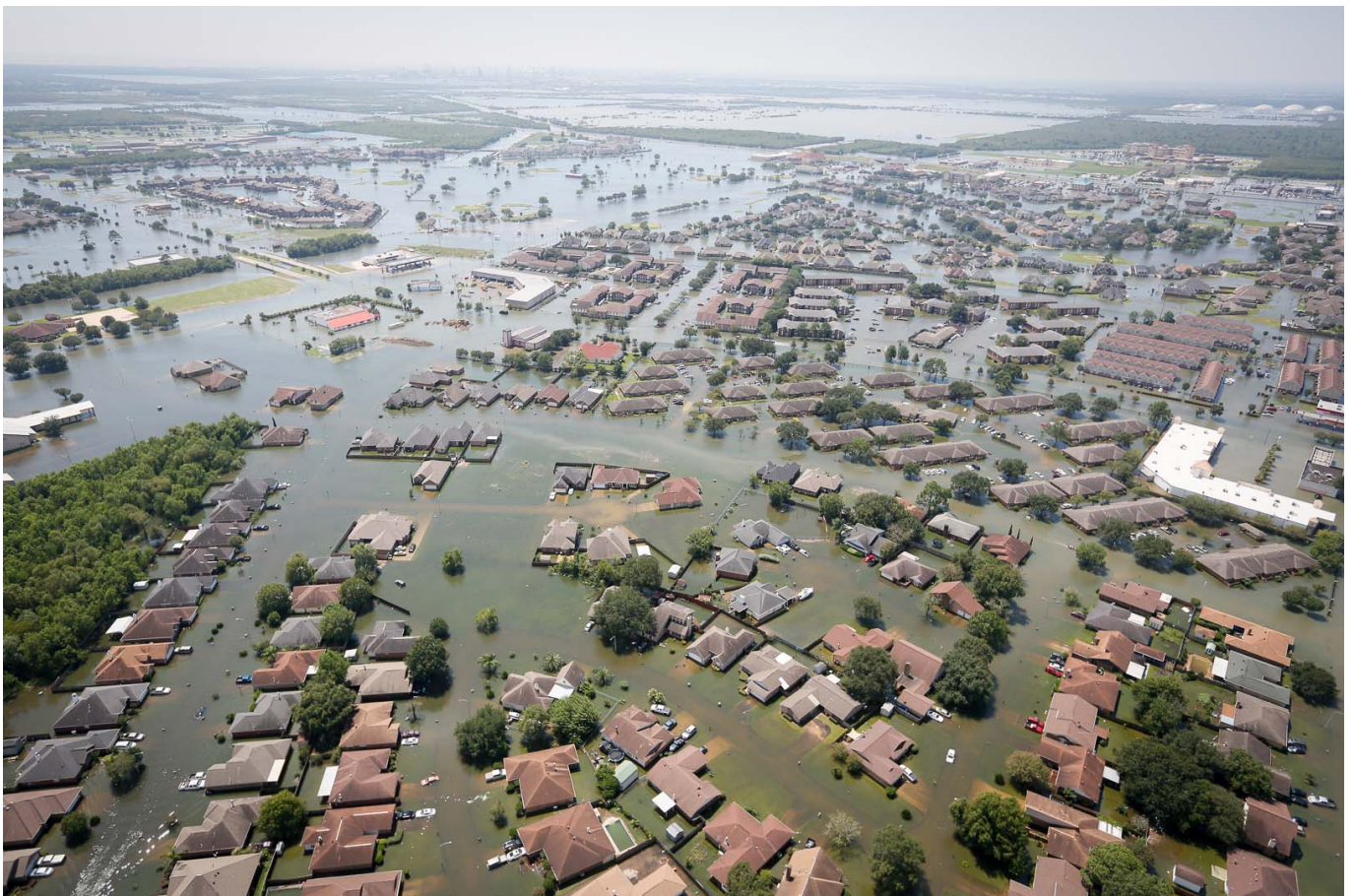
Hurricane Harvey flooded entire neighborhoods, 31. August 2017, (U.S. Air National Guard photo by Staff Sgt. Daniel J. Martinez, https://en.wikipedia.org/wiki/Hurricane_Harvey#/media/File:Support_during_Hurricane_Har
