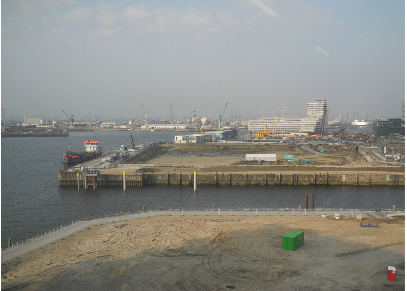
View along the River Elbe, Magdeburger Hafen and the temporary cruise ship terminals, Unilever Haedquarter and the Marco Polo Tower. (Photo by Dirk Schubert, 15.03.2015)
