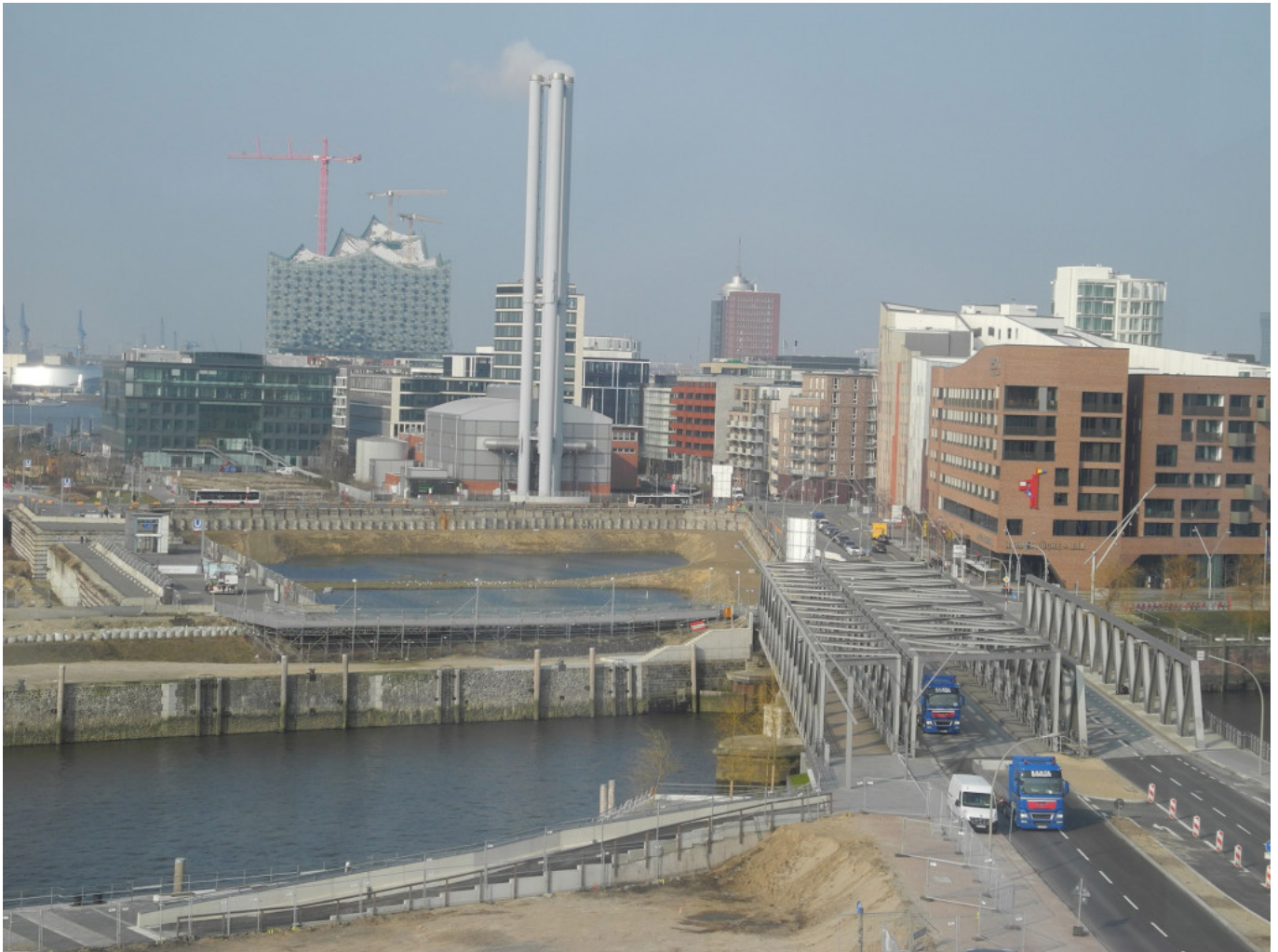
View over southern part of the construction site Überseequartier, the Elbphilharmonie in the background with a tower crane. (Photo by Dirk Schubert, 15.03.2015)
