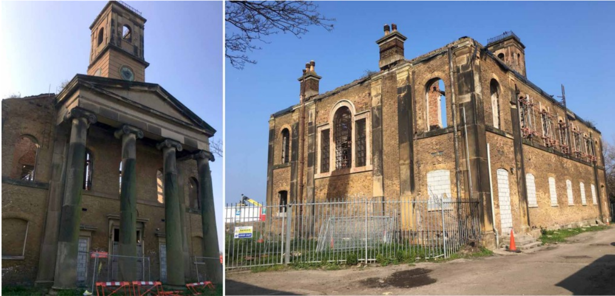
The Dockyard Church: the tetrastyle Ionic portico and the back. (Source: © Miki Fossati).
