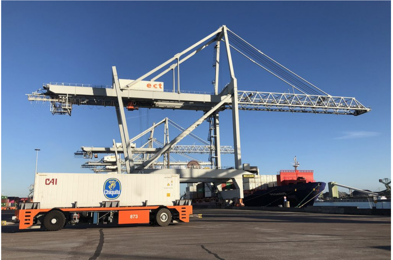
ECT container cranes and Automated Guided Vehicle-AGV system. (© Leon Willems, 2020; Source: Port of Rotterdam Authority).
