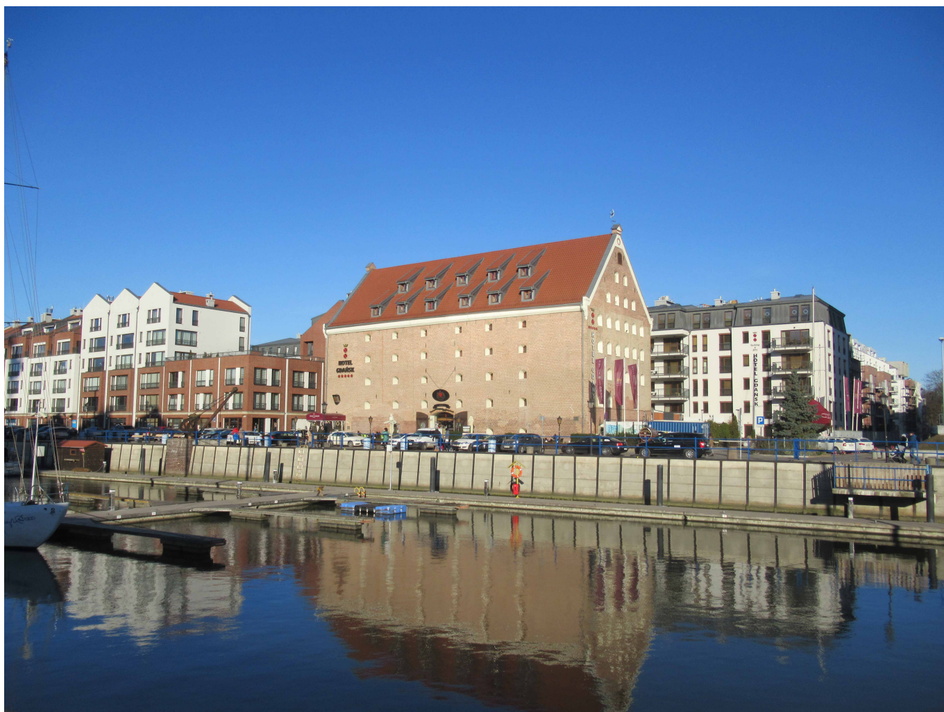
Granary building of the Renaissance origin - recently converted to the hotel and restaurant complex. Picture by P. Lorens. (fig. 9)
