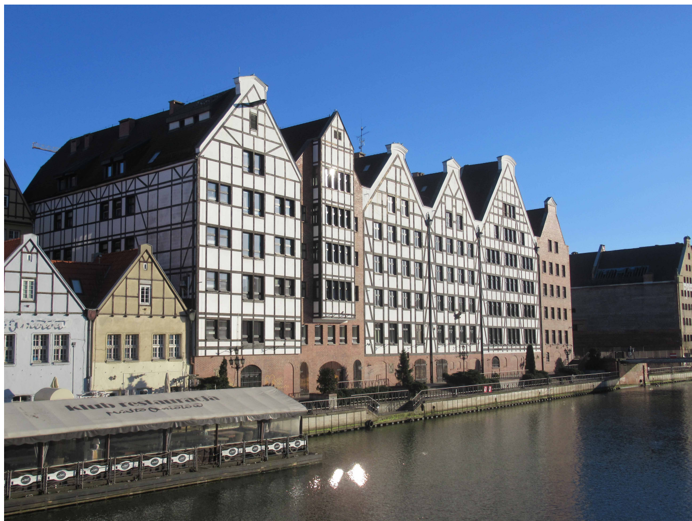
Introduced new buildings which shape and structure resemble the historic originals. Picture by P. Lorens. (fig. k)
