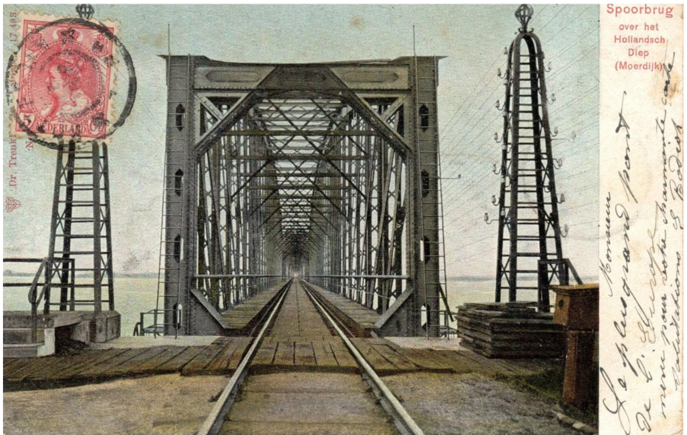
The industrial revolution eroded the romantic character of port cities, and instead encouraged awe for machinery. This Spoorbrug railway-bridge postcard has no trace of human beings. It shows the new use of iron and its capacity to span much larger distances than wood or stone. (© Source: Collection PortCityFutures).
