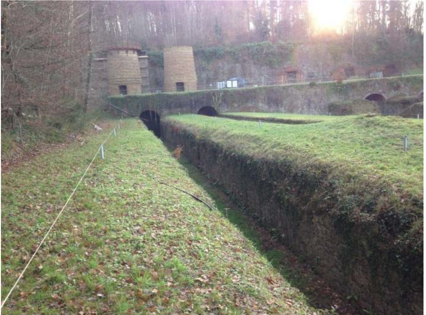
Iron Ore Loading tunnels IIWW. Normandie, France.
