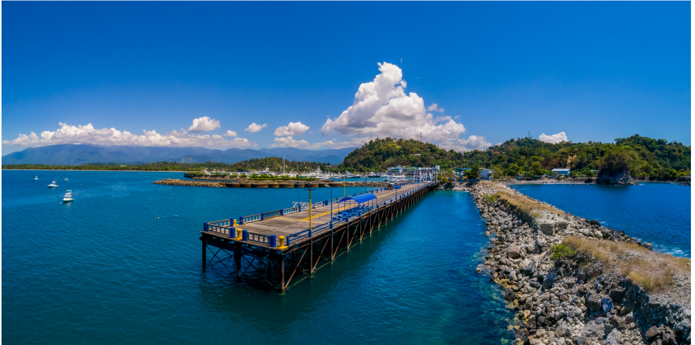
A port view of Quepos and the dock detail. (Source: INCOP)
