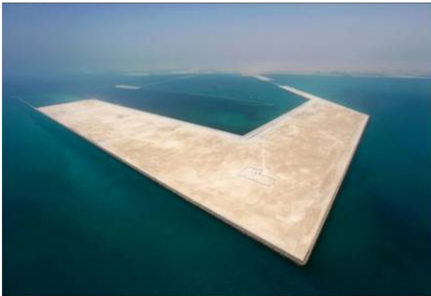
Khalifa Port. Fuente: https://www.bechtel.com/khalifa-port-and-industrial-zone.html
