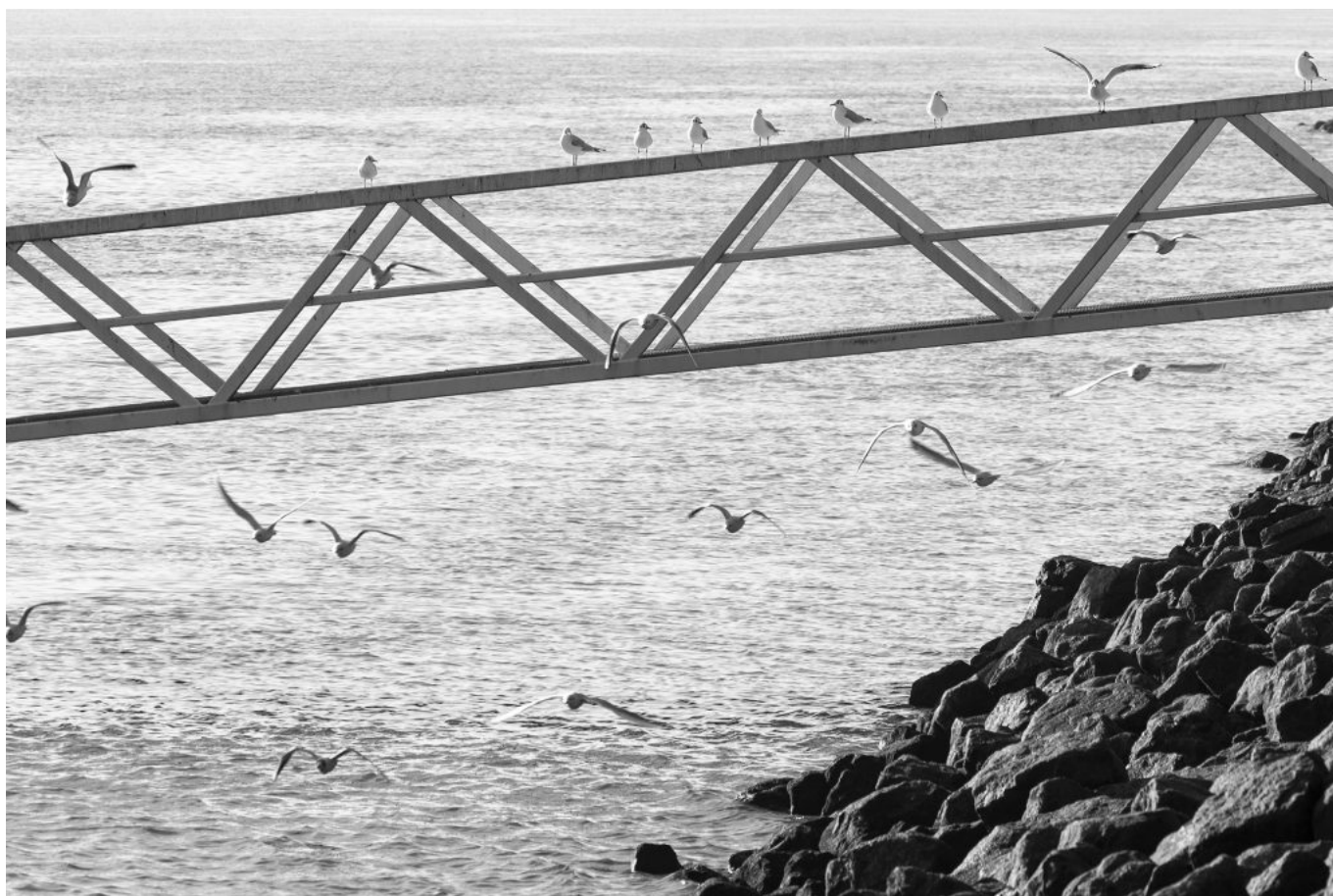
Water taxi pier ramp in the Maas. (© JGF|ph. Jacopo Gennari Feslikenian, 2019).
