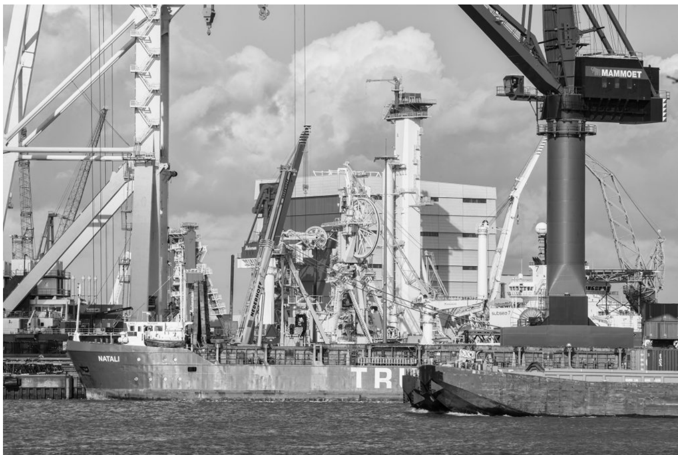
Wiltonhaven, view from the south bank of Neue Maas, Vijfsluizen - Schiedam. (© JGF|ph. Jacopo Gennari Feslikenian, 2017).
