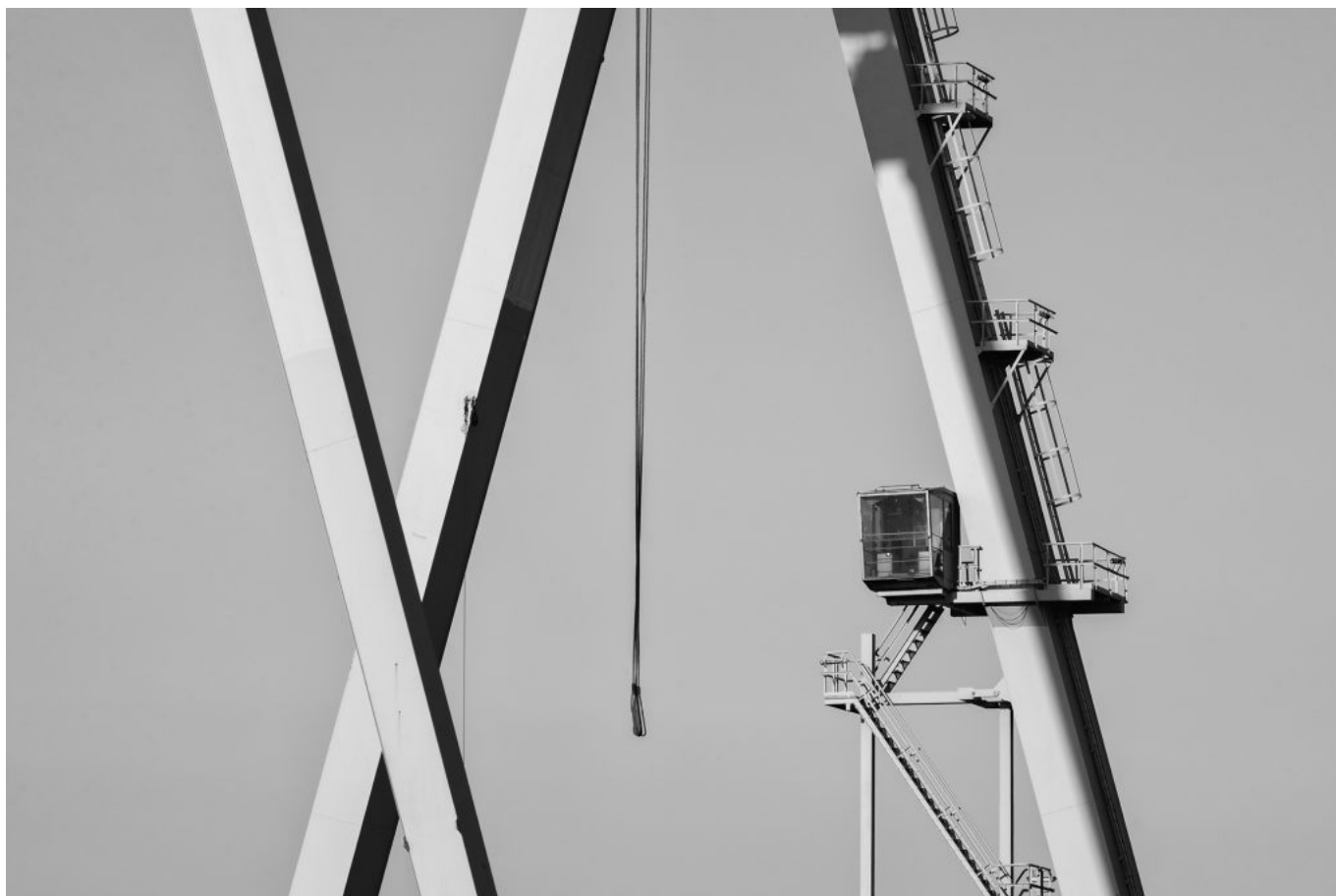
Cranes in Charlois Doklaan, Rotterdam. (© JGF|ph. Jacopo Gennari Feslikenian, 2017).
