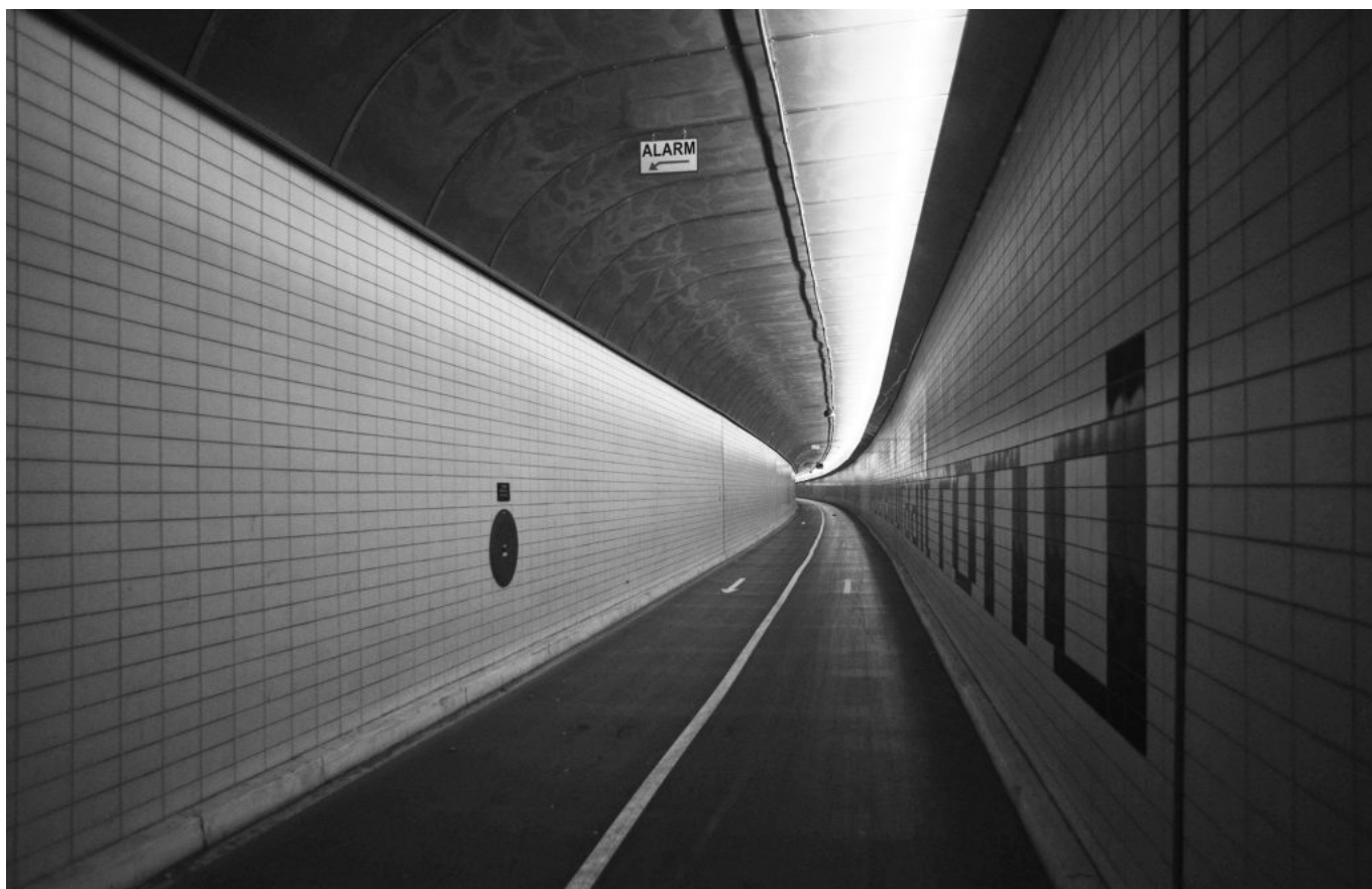
Cycling under the maas, Benelux Tunnel, Schiedam. (© JGF|ph. Jacopo Gennari Feslikenian, 2018).
