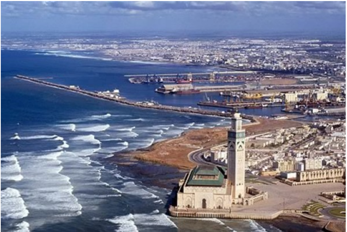
The site of the port of Casablanca.
