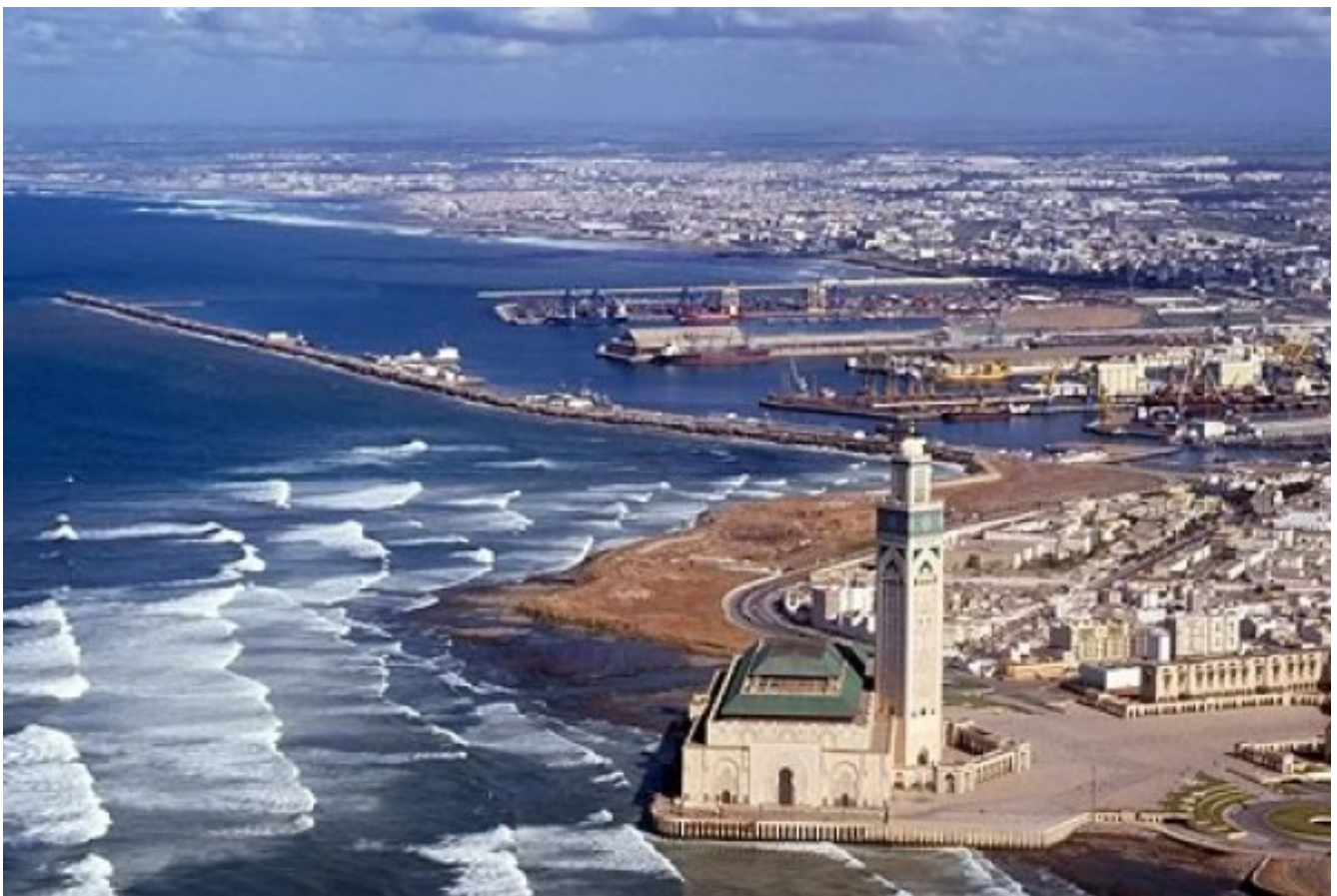
The site of the port of Casablanca.
