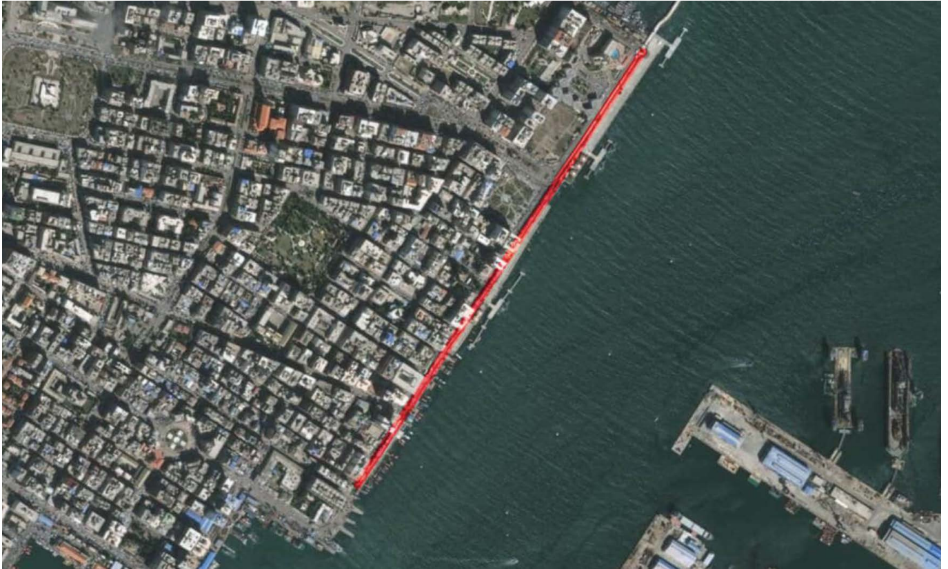
Elevated pedestrian promenade in Port Said (Ahmed Ades, 2017). Urban voids and resilience in Egyptian port-cities.
