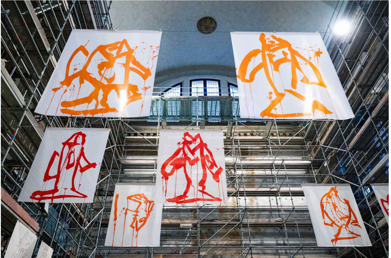
The church of San Lorenzo (left) and the Ocean Space project (right) in the recovered building. (© Enrico Fiorese)
