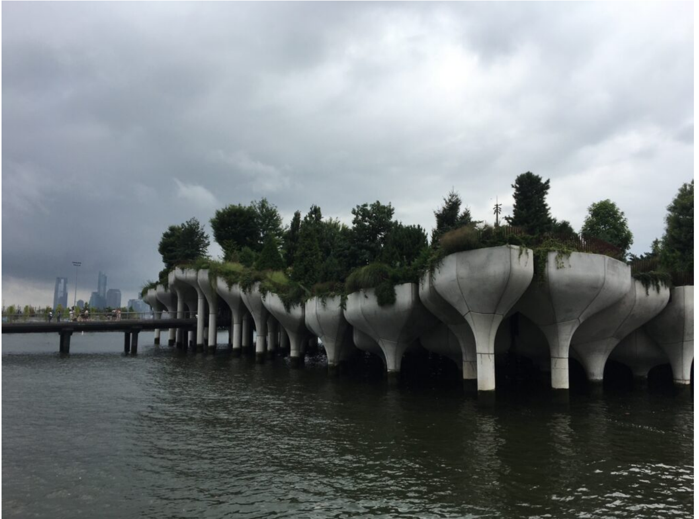
View of Little Island from Pier 57. (© Marta Moretti).
