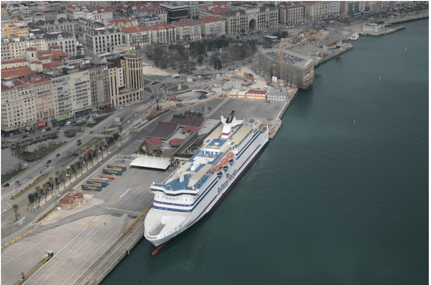
Passenger terminal and waterfront of the Port of Santander 2014. (Collection of the Port Authority of Santander. Photo: Foto Asturias S.L.)
