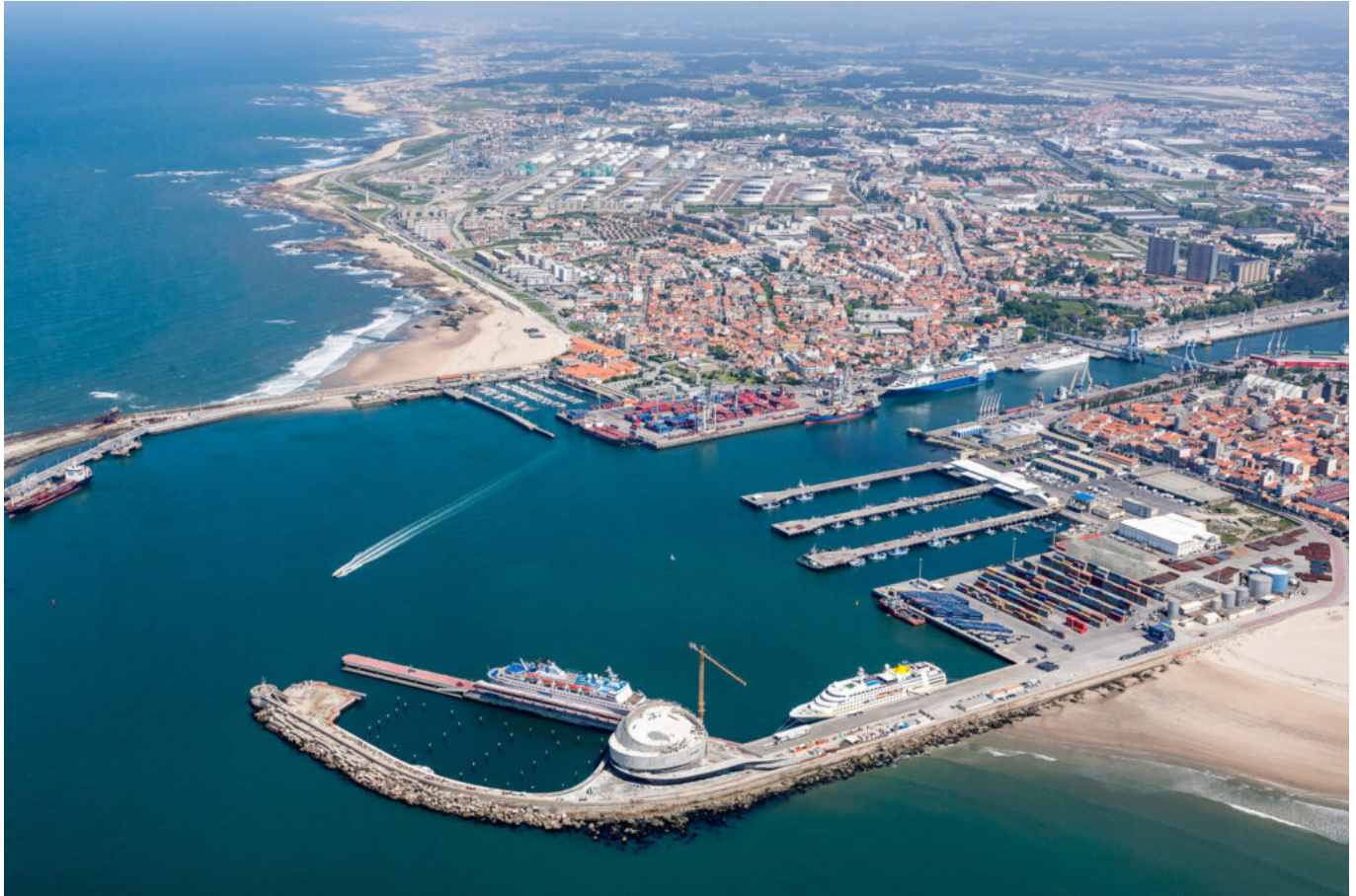
Aerial view of Port of Leixões and its remarkable cruise terminal. (© Matosinhos City Hall).
