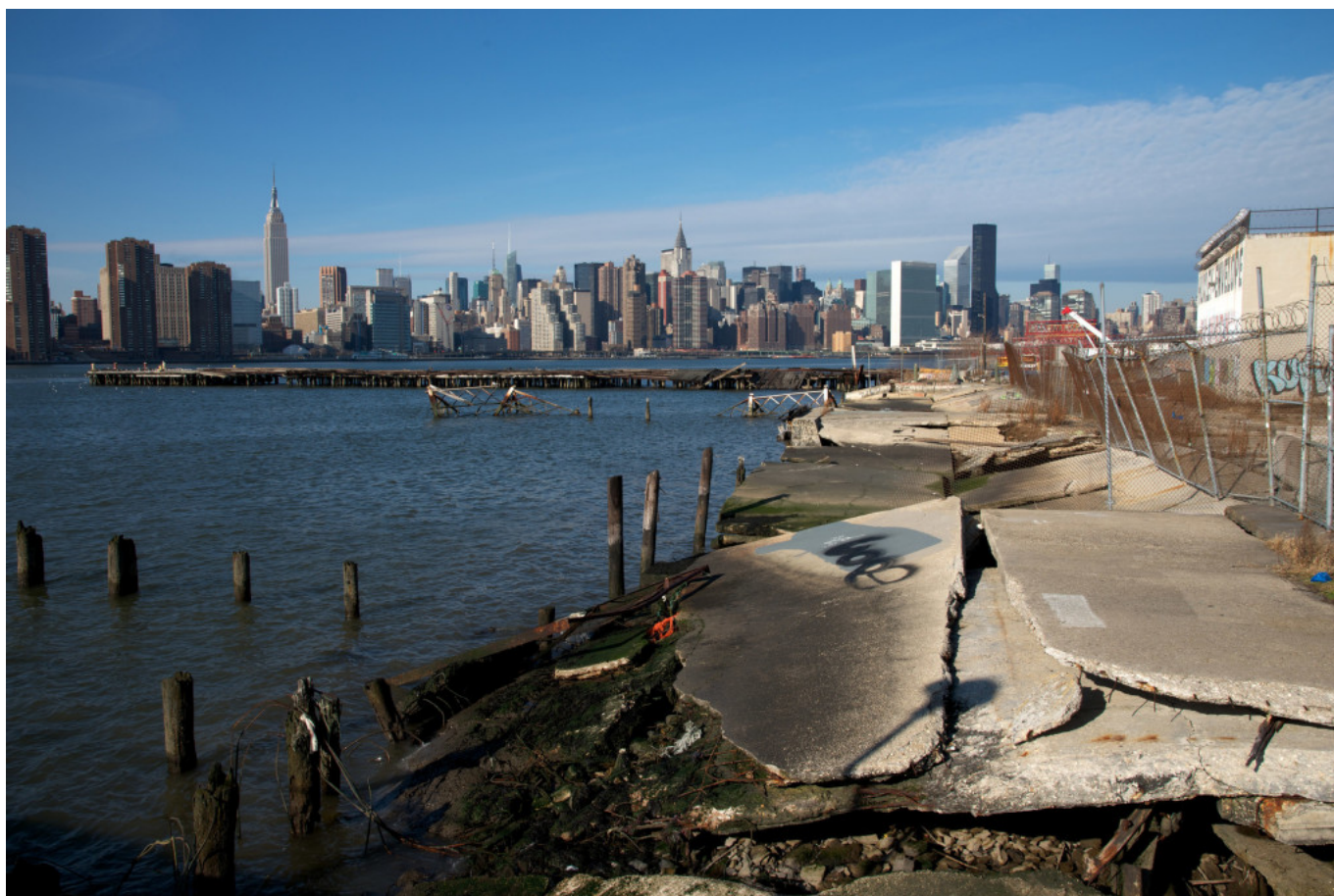
Abandoned piers in Greenpoint. Photo Copyright © Joan Alemany Llovera
