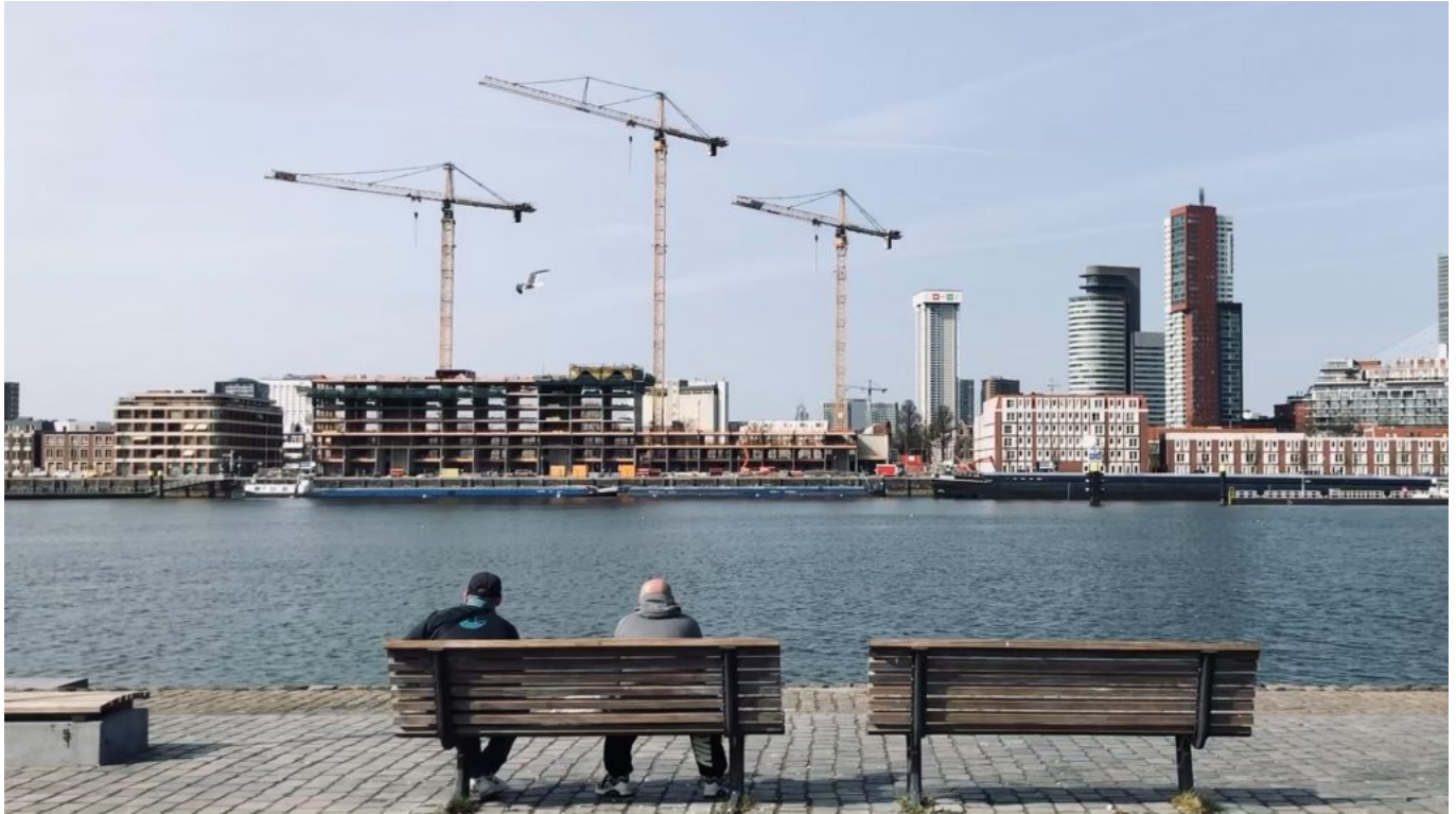
View on Maashaven and the redeveloping Katendrecht pier, Rotterdam. (© Maurice Harteveld, 2021).
