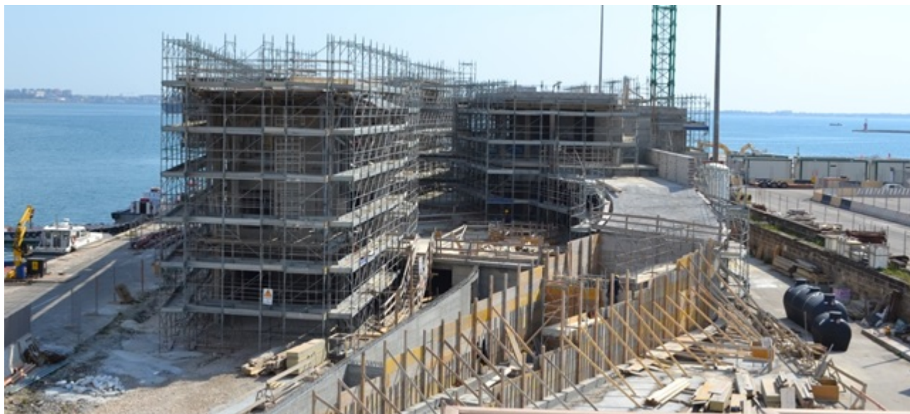
The Falanto Port Service Center (as is).
