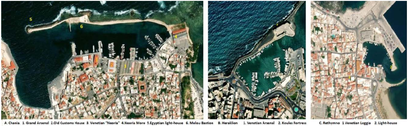
Heritage port structures in Chania, Heraklion and Rethymno. (Composed by the author based on aerial pictures from carto.com)
