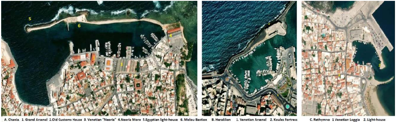
Heritage port structures in Chania, Heraklion and Rethymno. (Composed by the author based on aerial pictures from carto.com)
