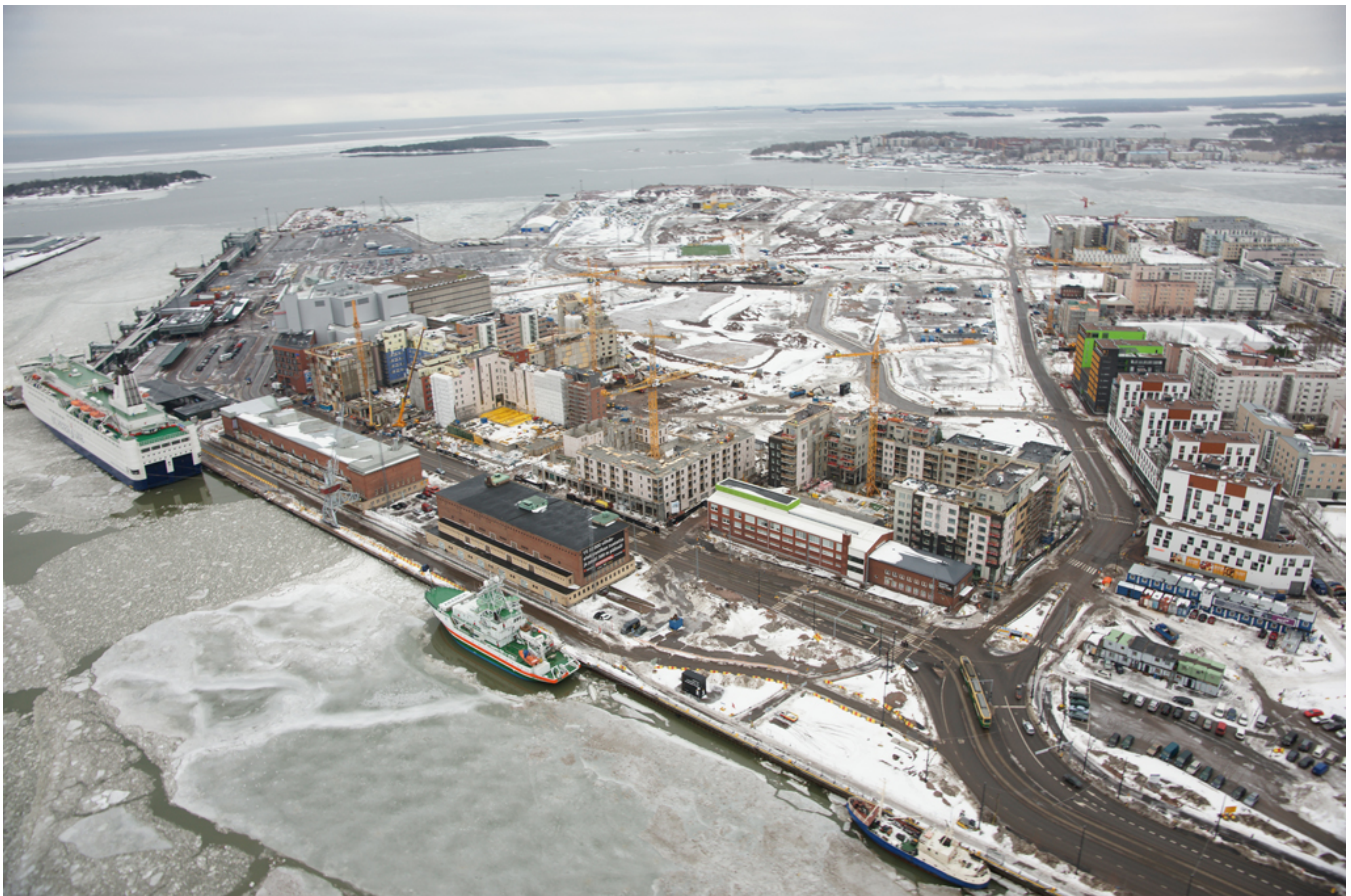
Jätkäsaari in January 2013. Construction has begun by the city centre.
