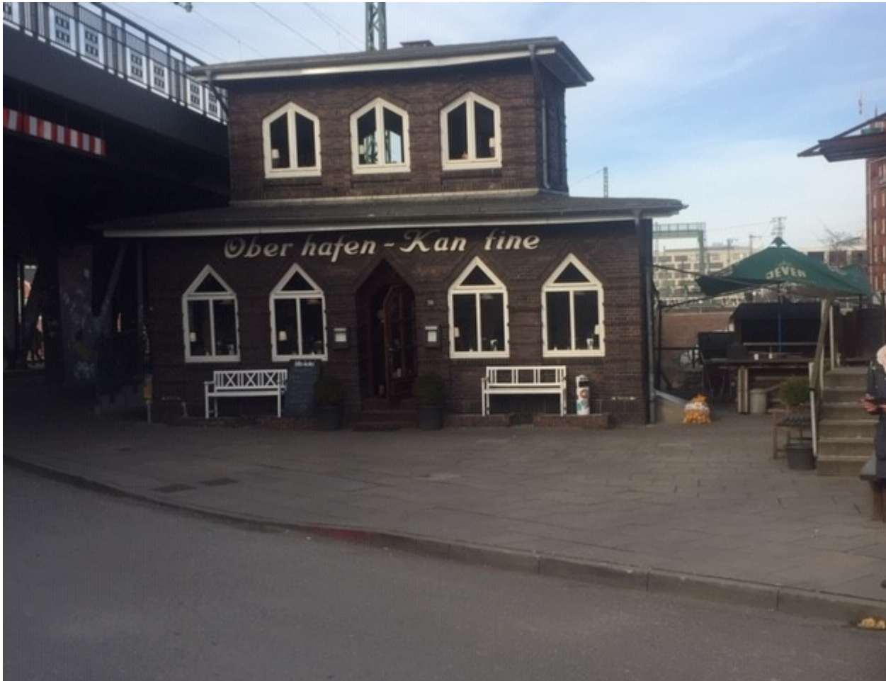
Oberhafenkantine, Former canteen for dockers. (Dirk Schubert)
