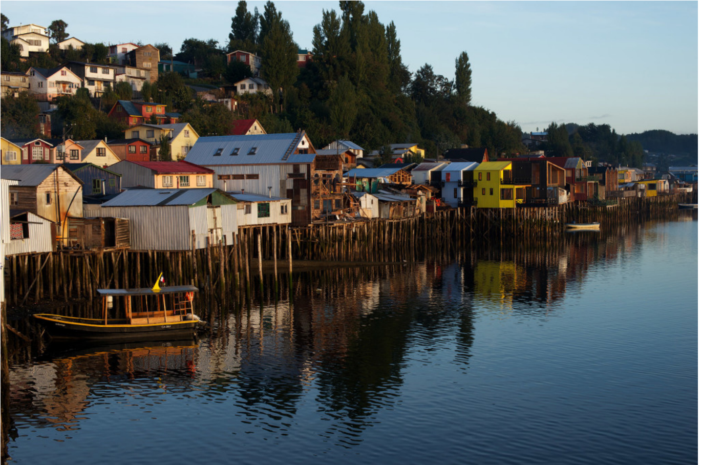
Renovation of palafitos (houses on the water) in Castro. (© Joan Alemany)
