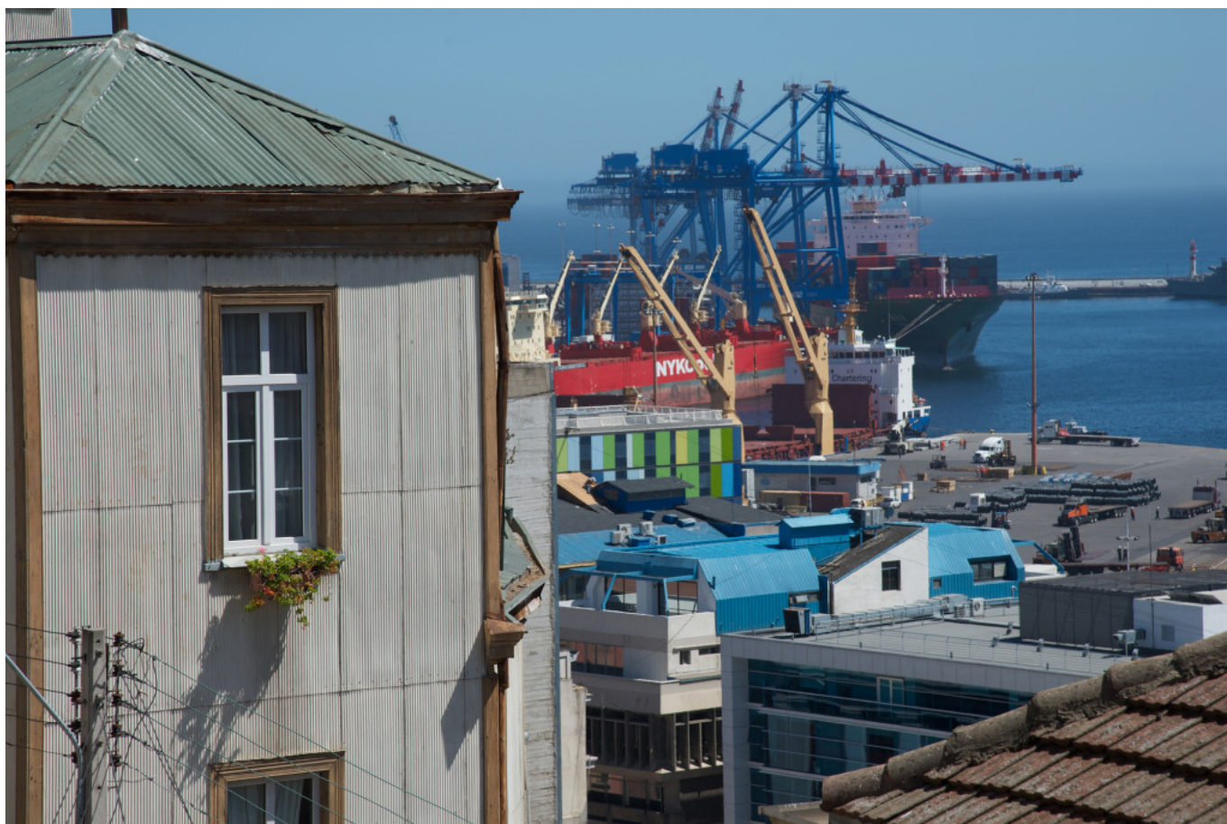
Permanent presence of the port in Valparaiso. (© Joan Alemany)
