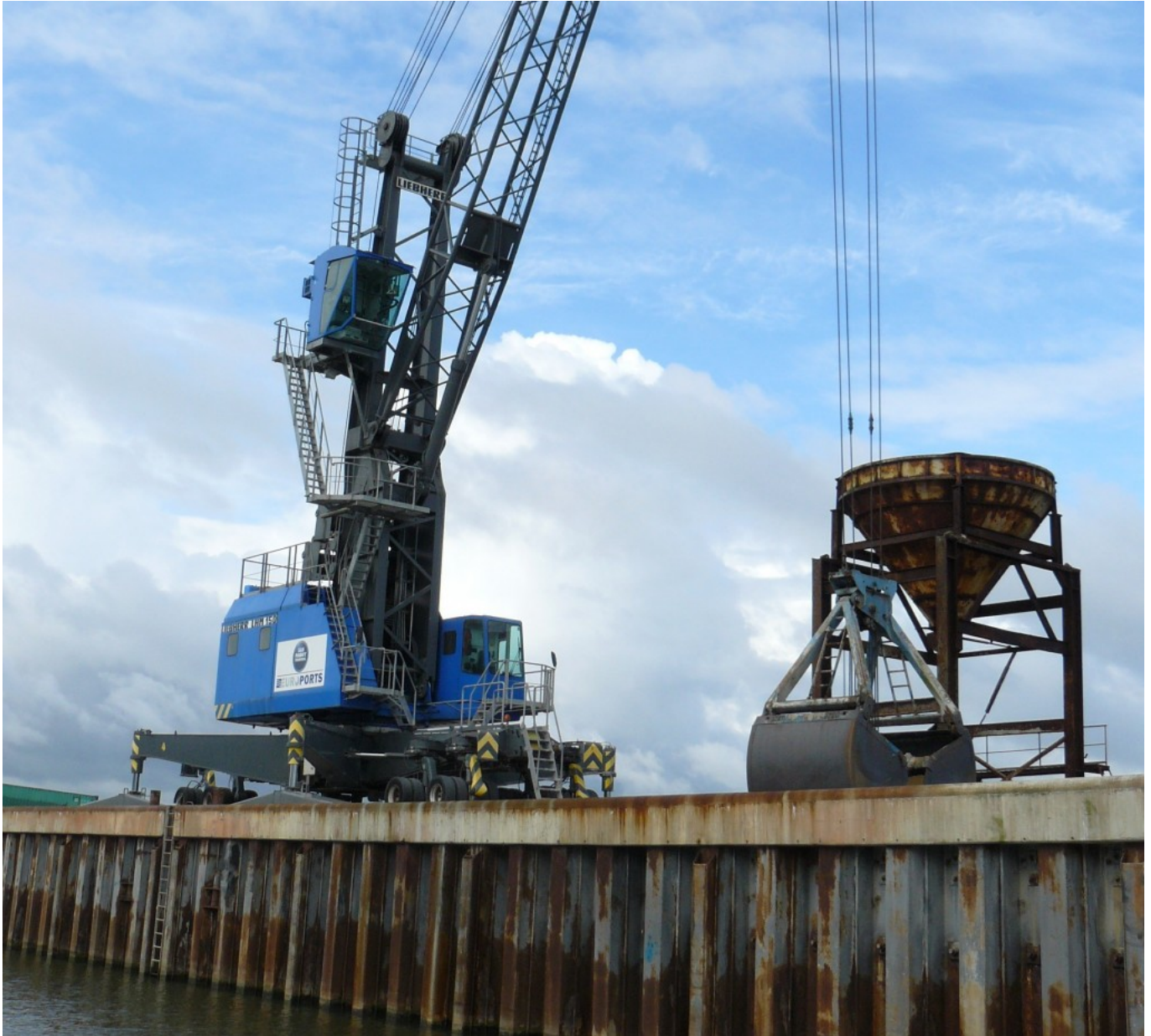
The capacities of French inland ports are widely underutilized. (Photo © Pierre Gras)
