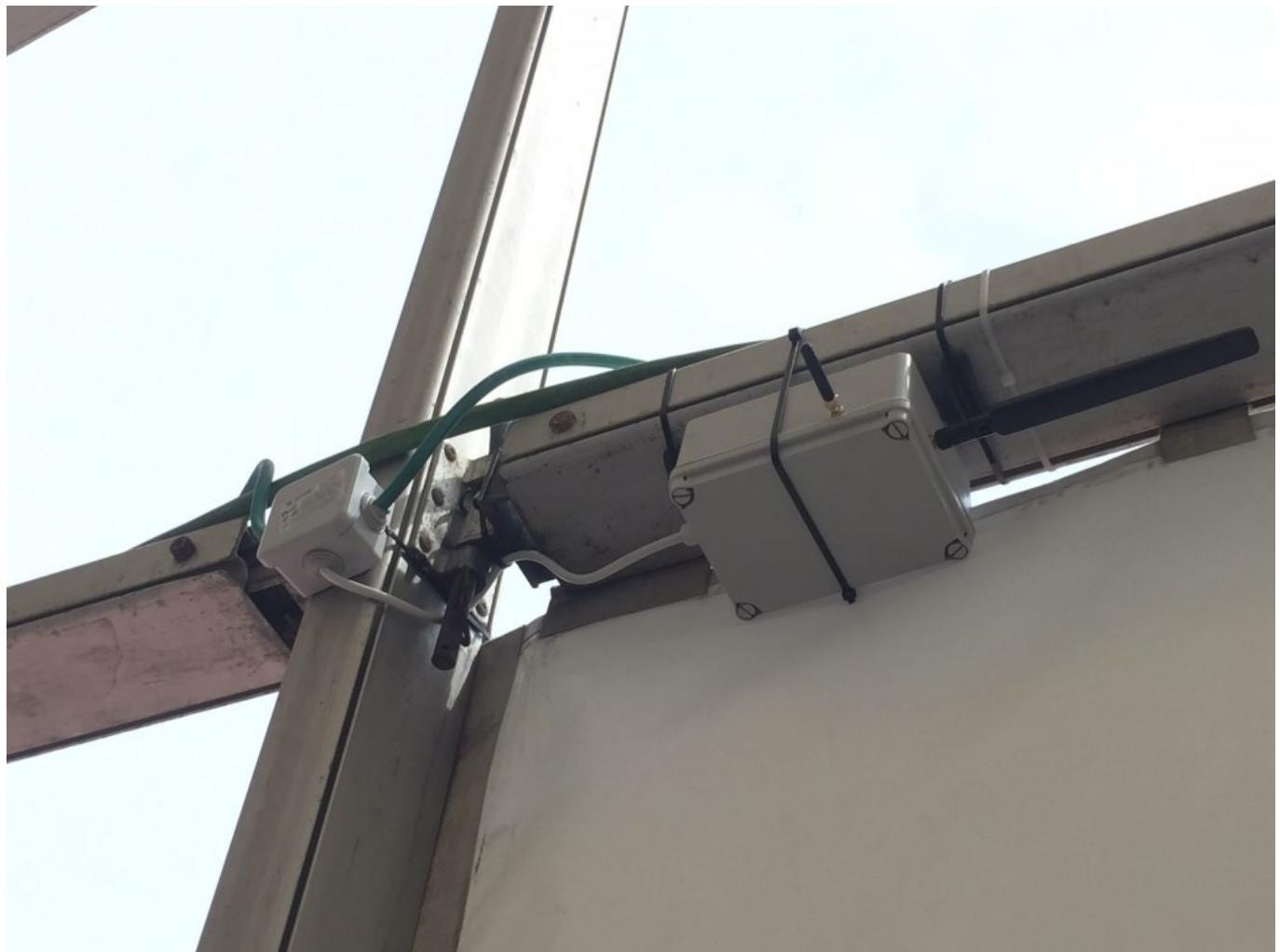
*WiFi sensors installed in the cruise terminal. (Source: Fundación Valenciaport, 2021).*
