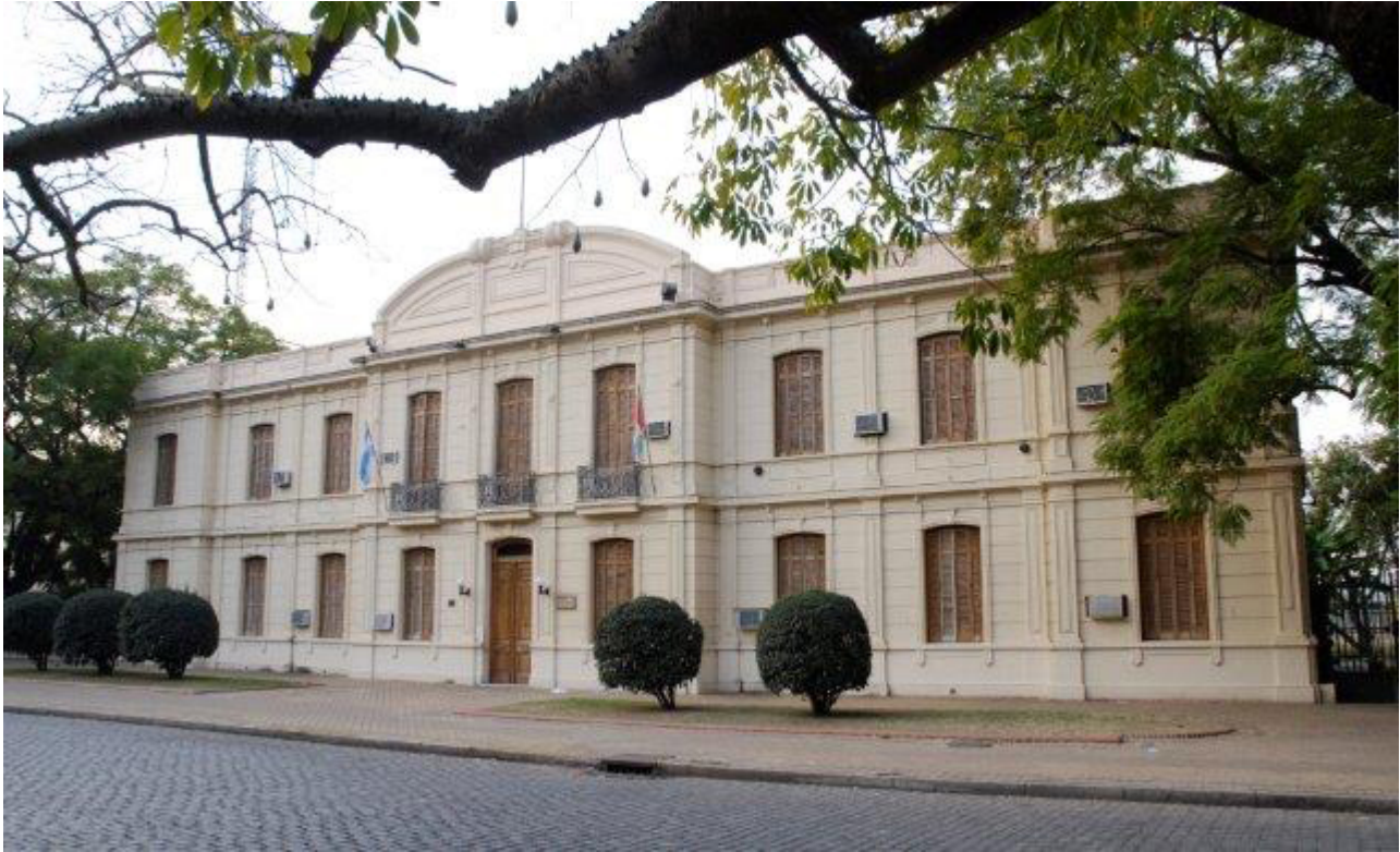
Building where the Administrator Entity of the Port of Rosario has its headquarters. ENAPRO Press Photography.
