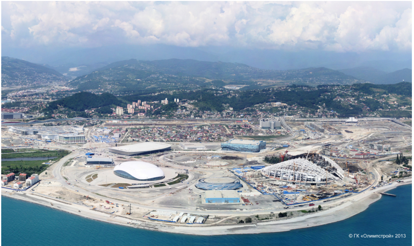
The yards in the Olympic Park under construction in Sochi. (© Olympstroy)
