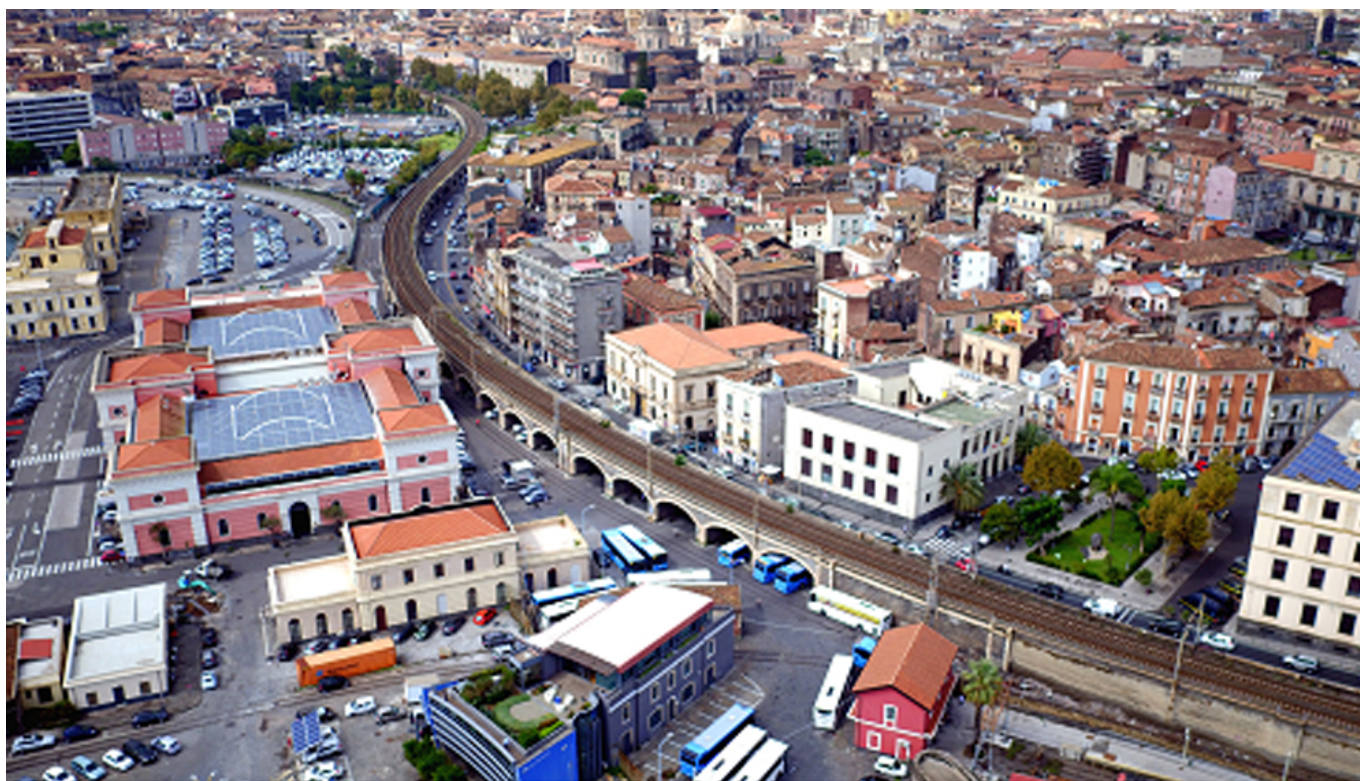
Harbour area between old and new constructions. (image courtesy of engineer Lentini, manager of the technical area Authority of Harbour Systems in Eastern Sicily)
