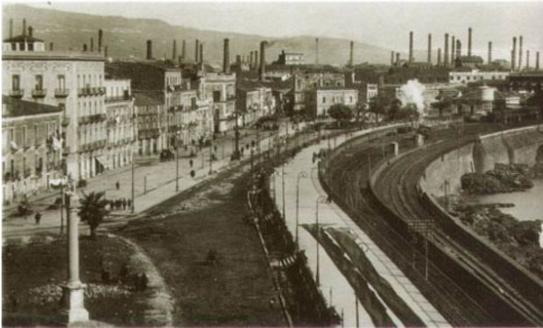
The early 1900s, railway hub and chimney stacks along the coast.
