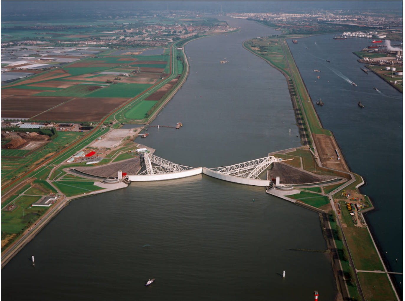
The New Waterway facing east with a closed Maeslantkering, the flood barrier in the New Waterway that was finished in 1998. (Source: Image repository Rijkswaterstaat / Afdeling Multimedia Rijkswaterstaat; https://beeldbank.rws.nl/MediaObject/Details/334490/ ).
