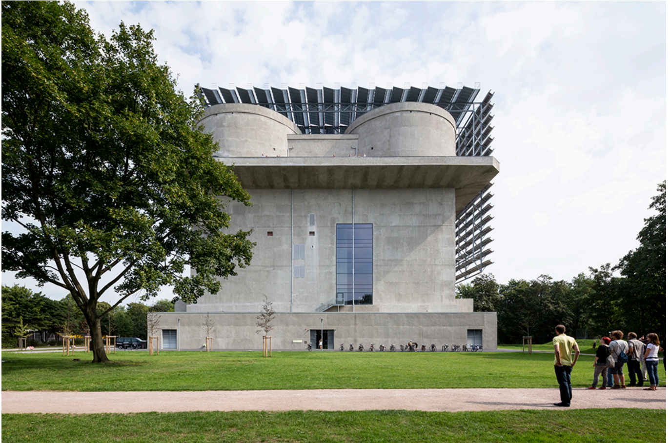
Energy Bunker: a war relic becomes a power station and energy reservoir.
