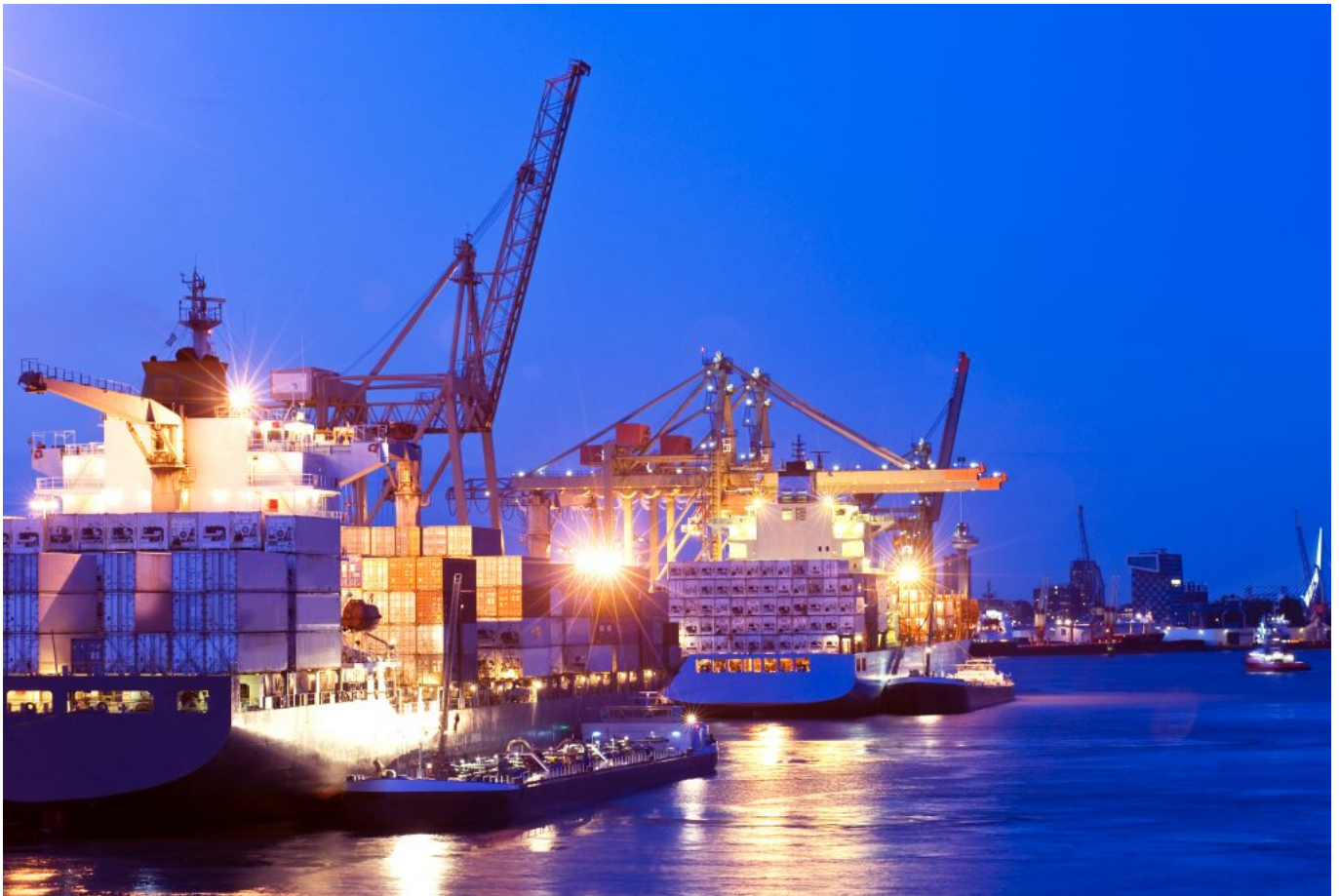
Port Facility. Activity of loading and unloading of container ships. (Source: INDRA Sistemas).
