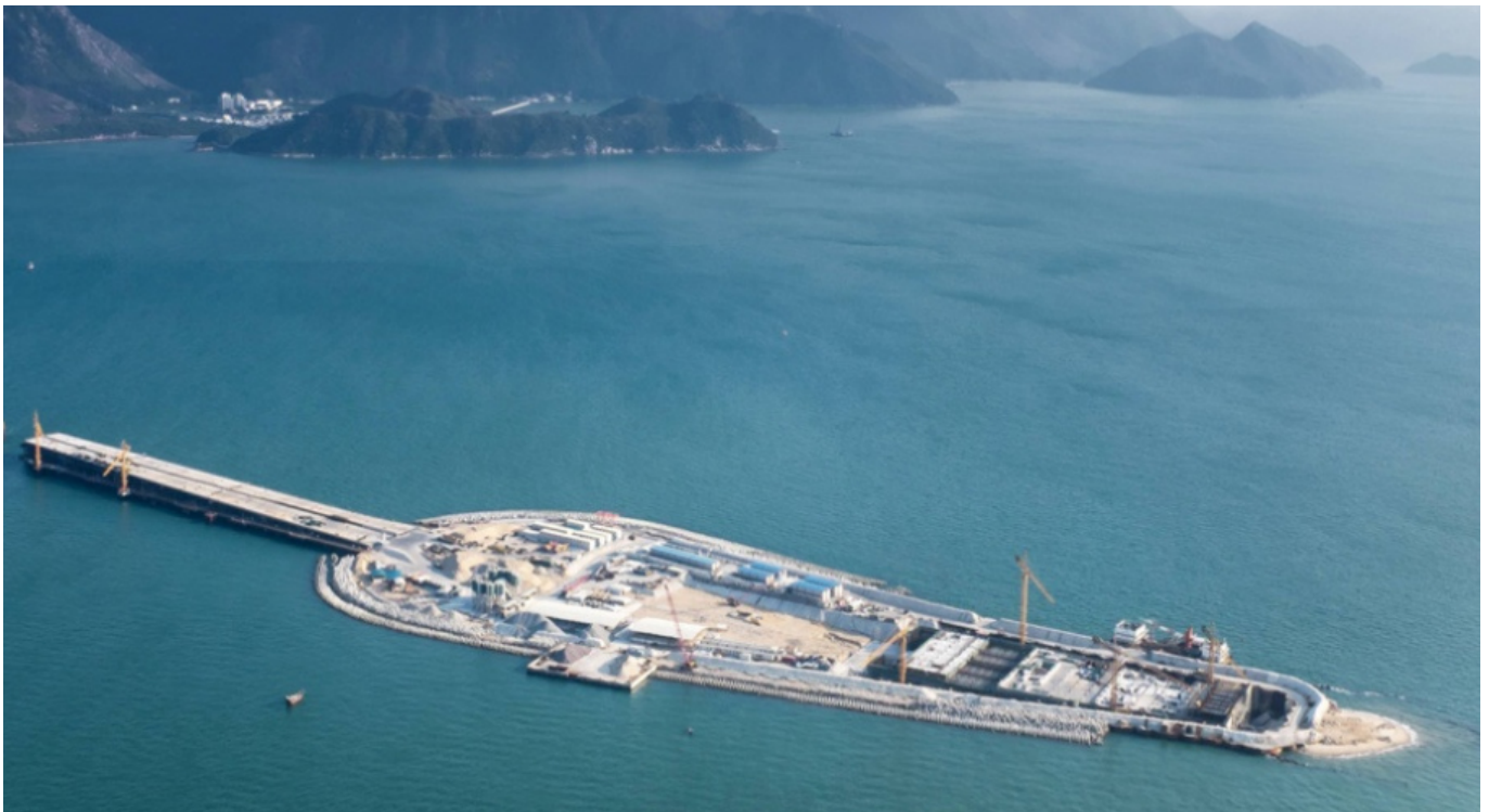
The Hong Kong-Zhuhai-Macau Bridge and the artificial island under construction.
