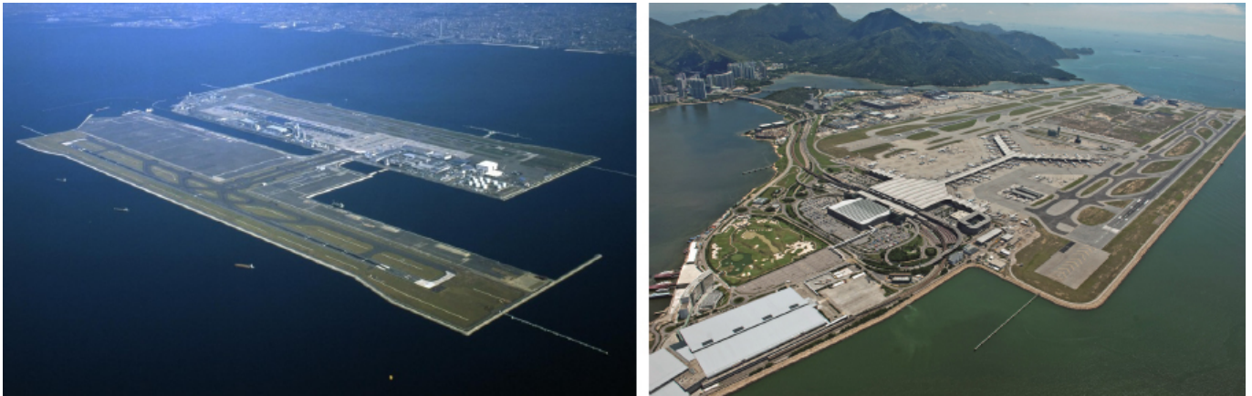
The international airports of Kansai (left) and Hong Kong (right) realized on artificial islands.
