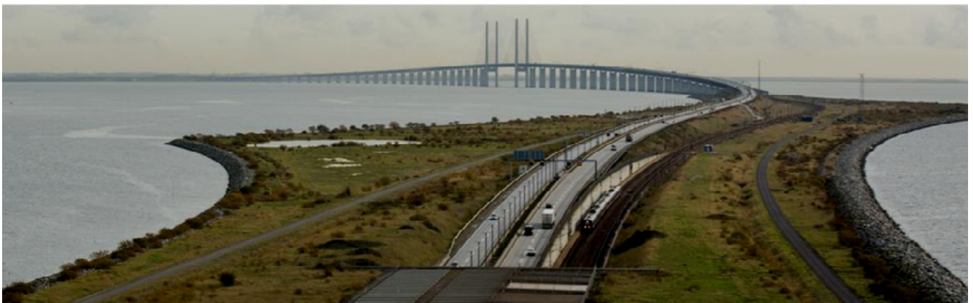
Integral part of the bridge that connects Denmark and Sweden, Peberholm is a small artificial island overlooking the strait of Oresund.
