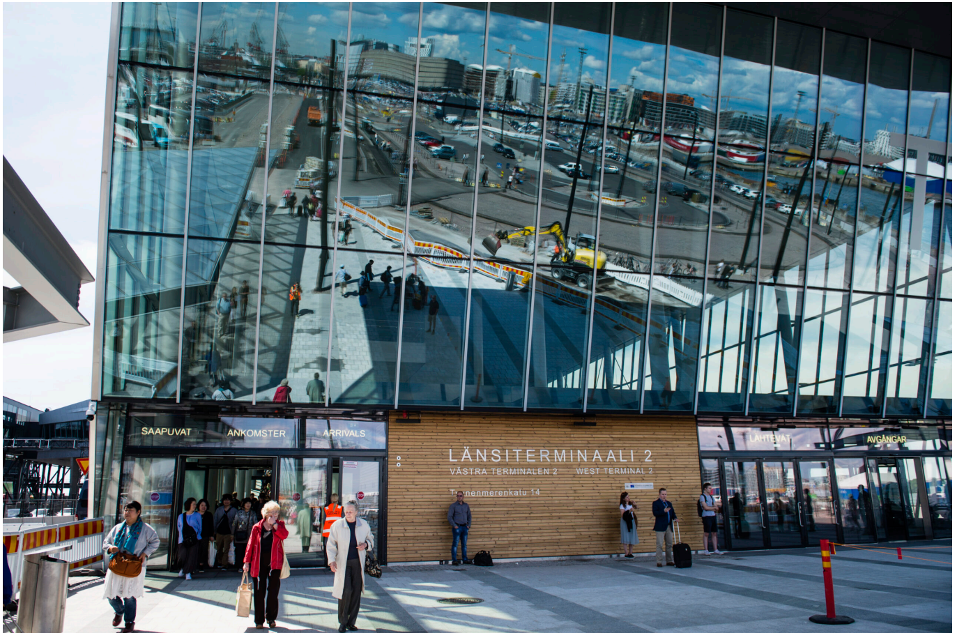
West Terminal at the Port of Helsinki. (© Port of Helsinki).
