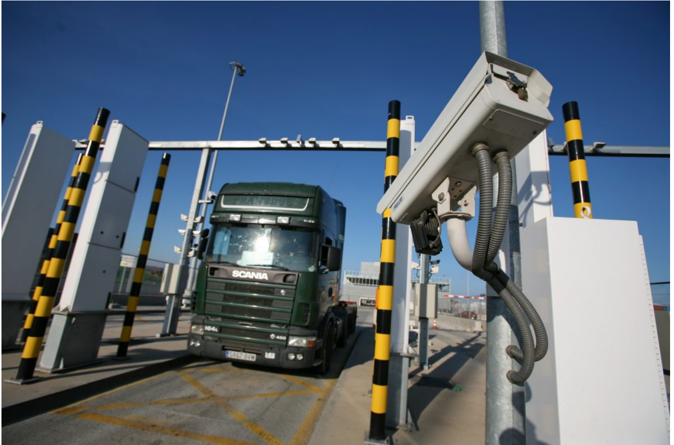
OCR of entry at the land access door to BEST. (© Barcelona Europe South Terminal - BEST).
