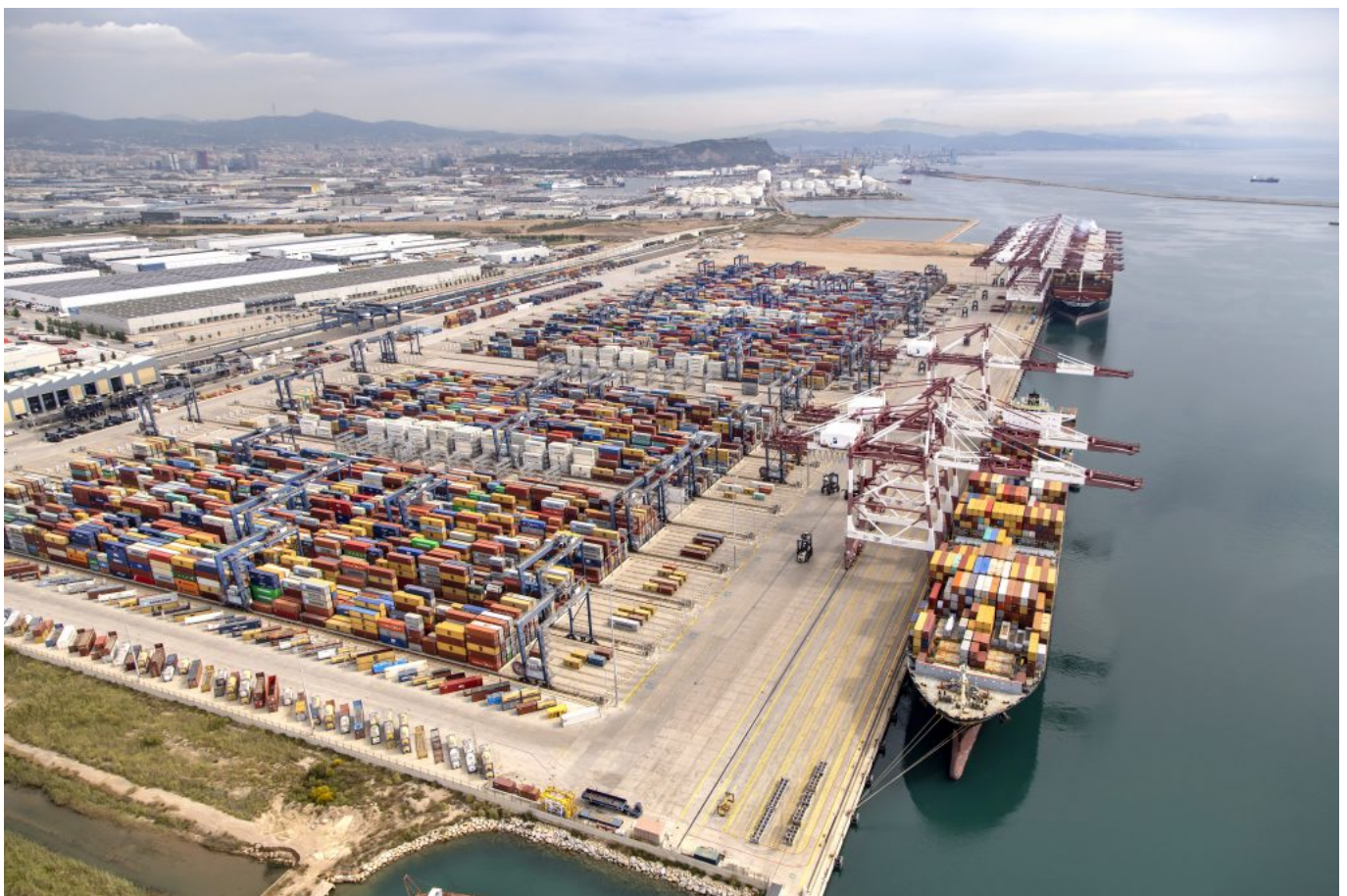
Aerial view of the BEST terminal. In the background the port and the city of Barcelona. (©
